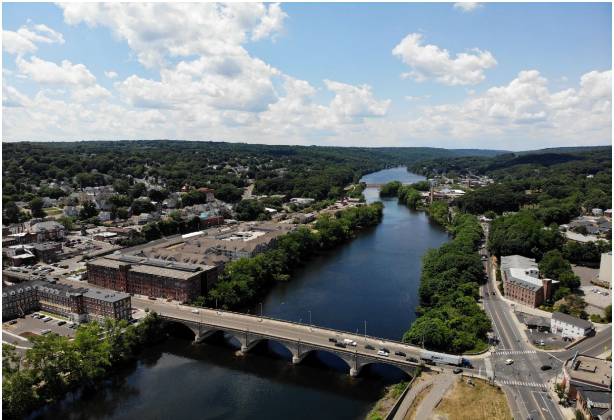
Aerial image above the Derby-Shelton Bridge, 2023
