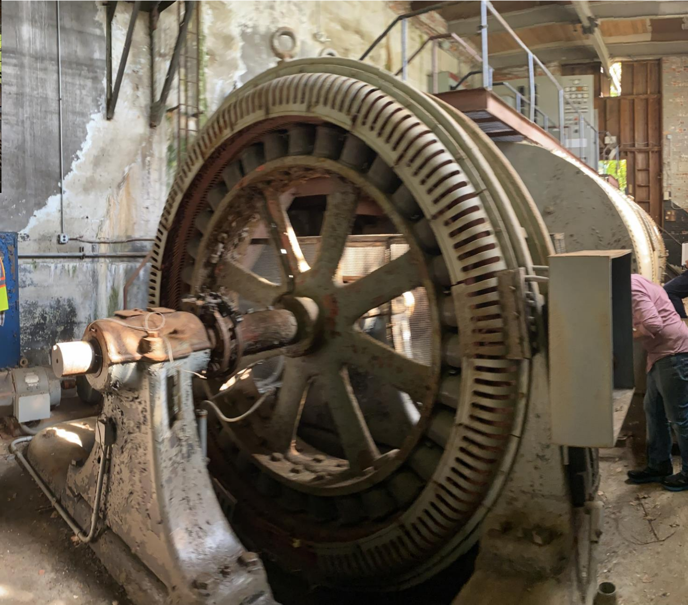
Turbine and Turbine housing (note pully system on ceiling I-beam)
