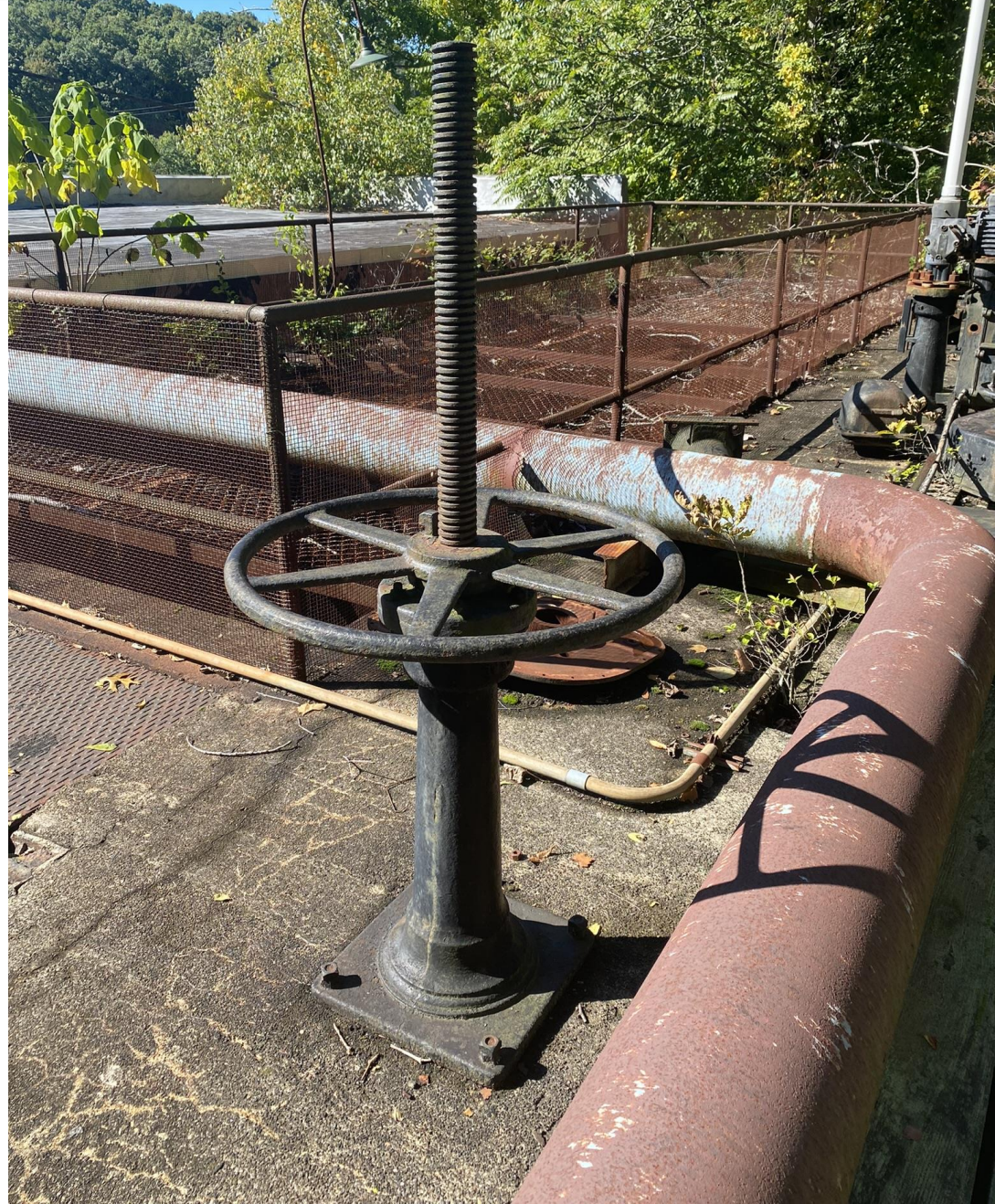
1 manual sluice gate and 3 mechanical sluice gates (it is unknown if they are operable)
