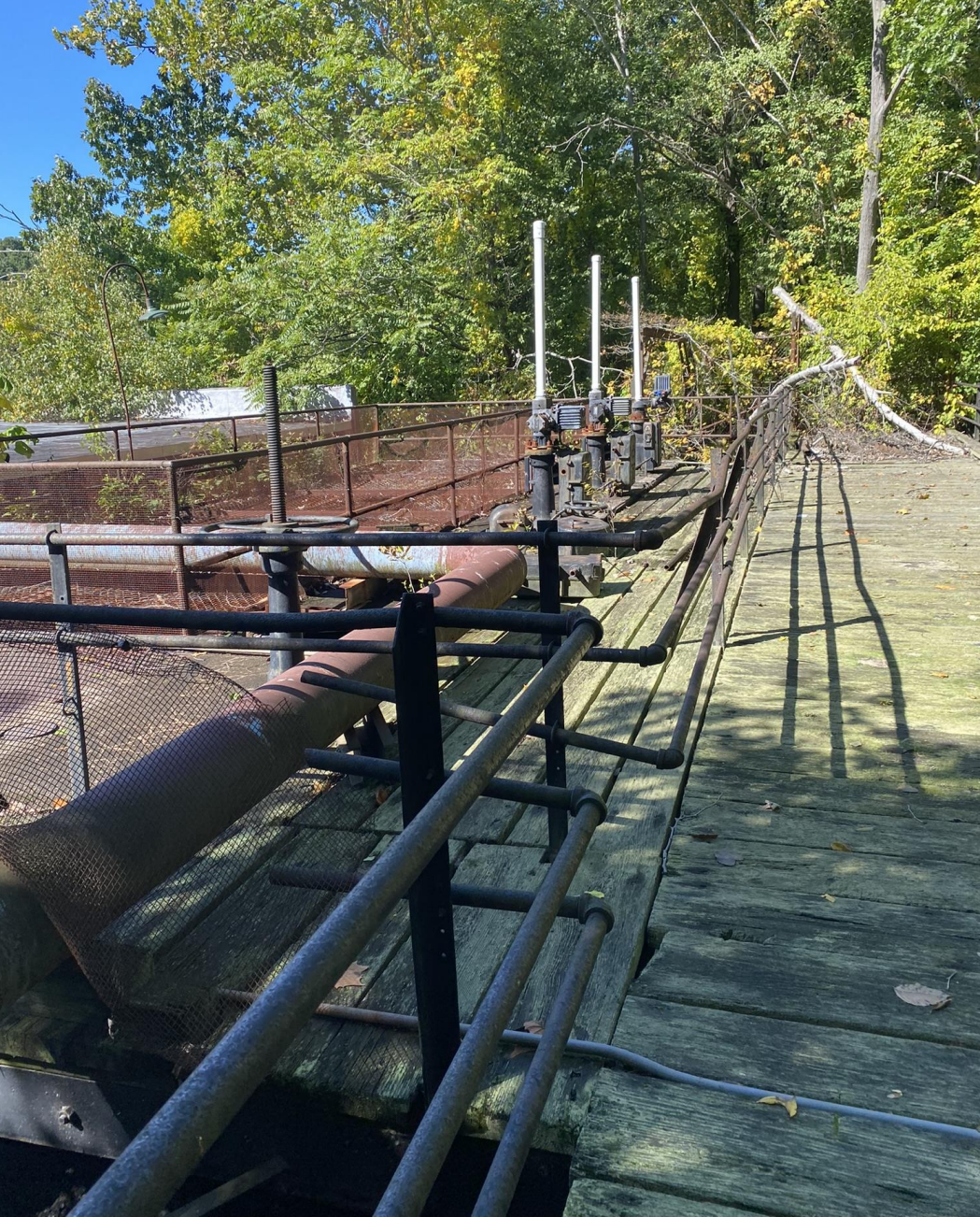
1 manual sluice gate and 3 mechanical sluice gates and wooden operating platform in poor condition
