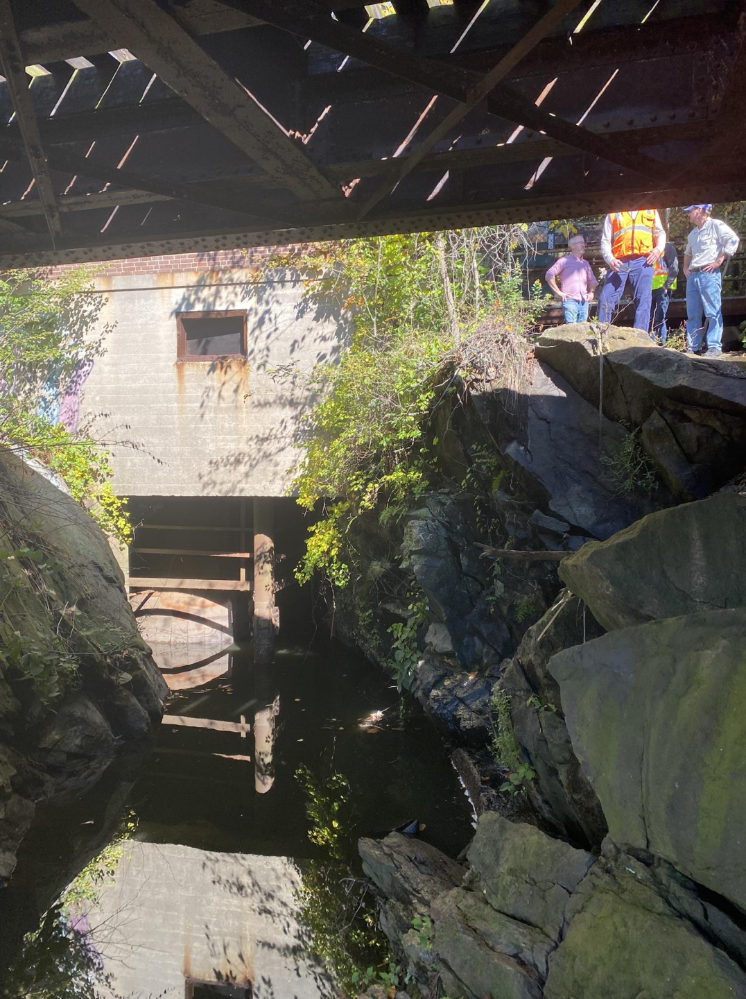
Turbine outlet pipe/riser visible beneath building (photo taken from underneath railroad bridge)
