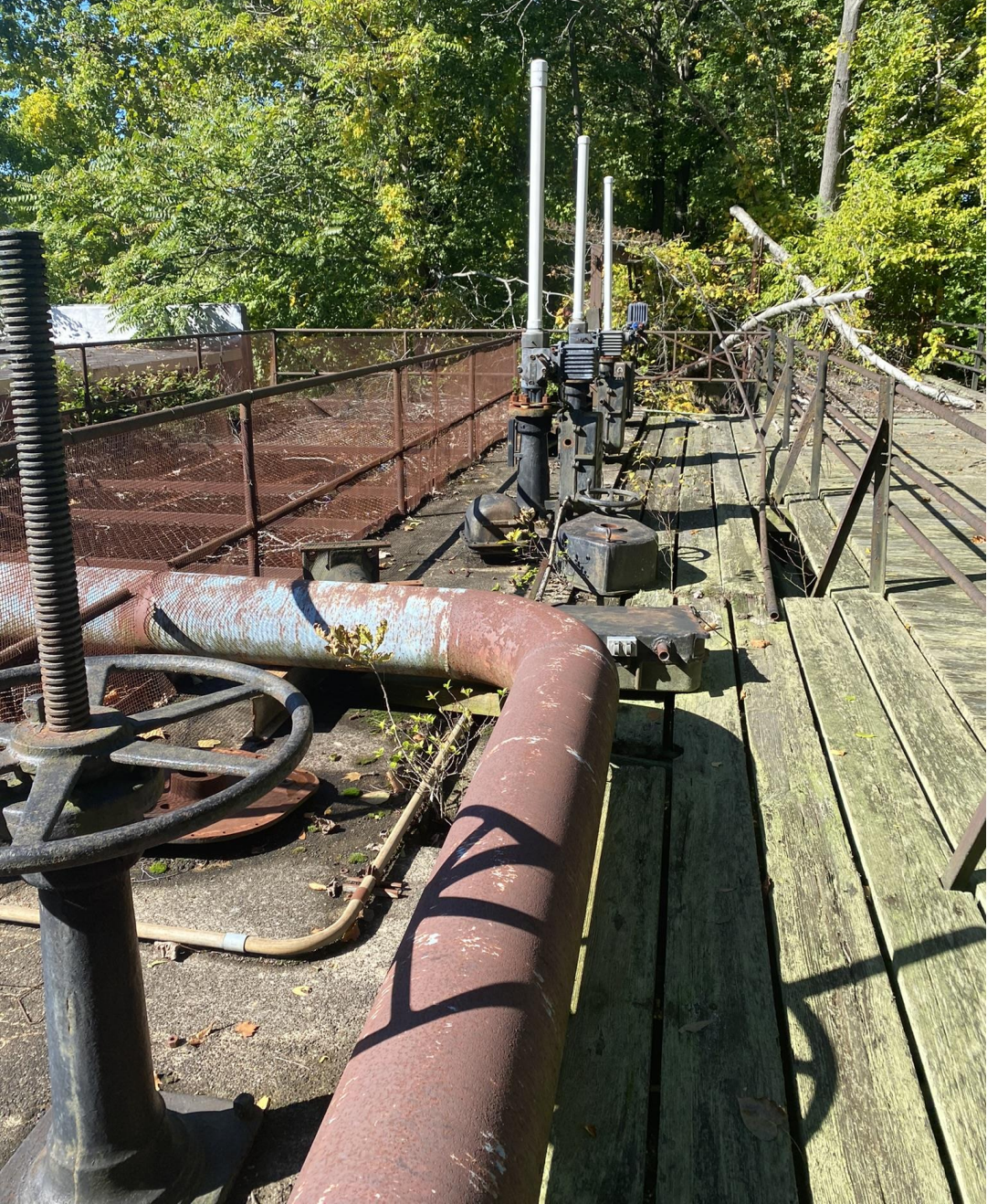
1 manual sluice gate and 3 mechanical sluice gates (it is unknown if they are operable)
