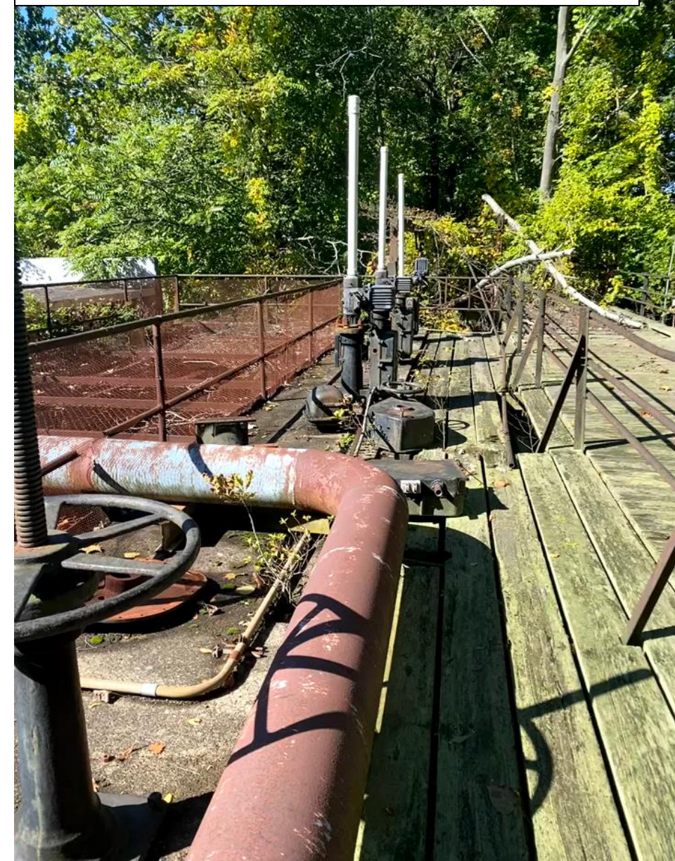
1 manual sluice gate and 3 mechanical sluice gates and wooden operating platform in poor condition
