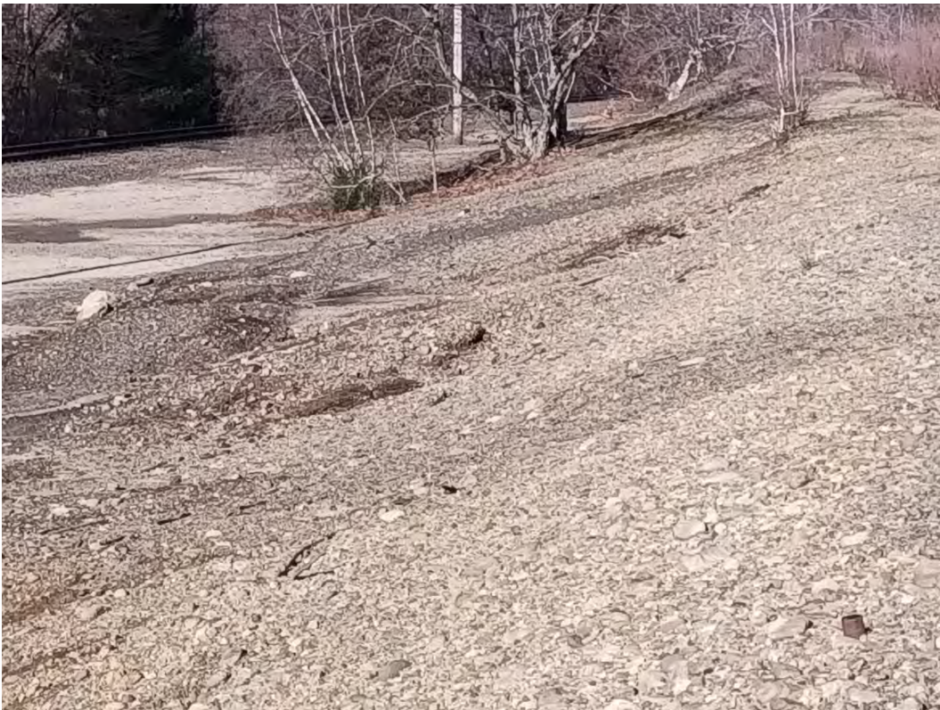
Photo 21. View of Outboard Slope. Note Presence of Silty Sand with Railroad in Background
