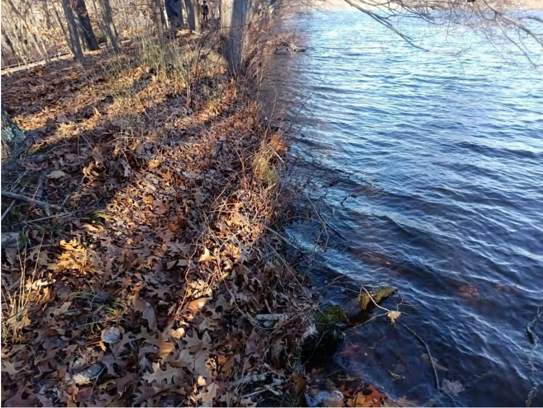
Photo 15. View of Inboard Slope. Note Near Vertical Bank and Lack of Riprap Armoring
