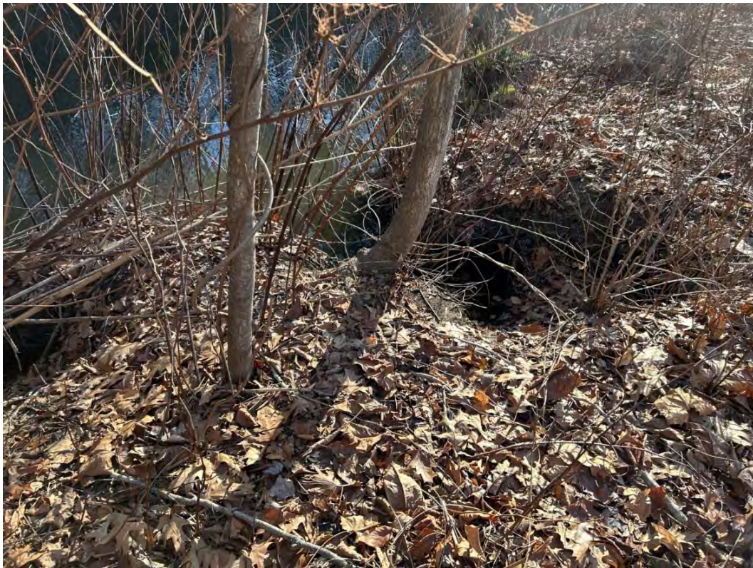
Photo 14. View of Inboard Slope. Note Presence of Woody Vegetation and Evidence of Rodent Burrow
