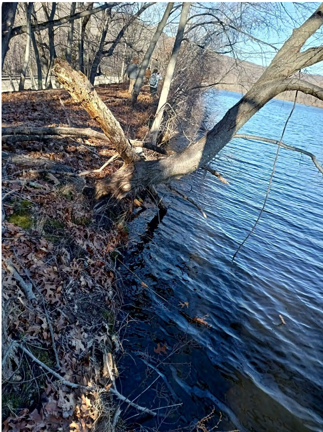
Photo 17. View of Trees Overhanging inboard slope
