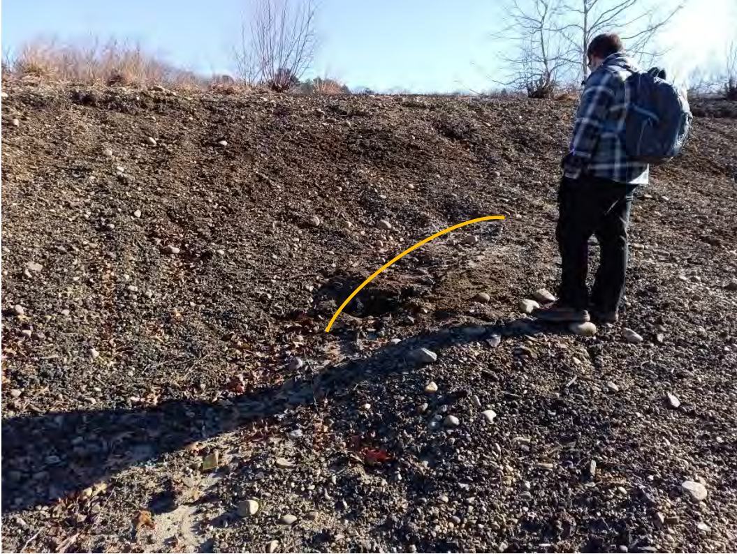
Photo 24. View of Outboard Slope. Note Apparent Shallow Slope Failure
