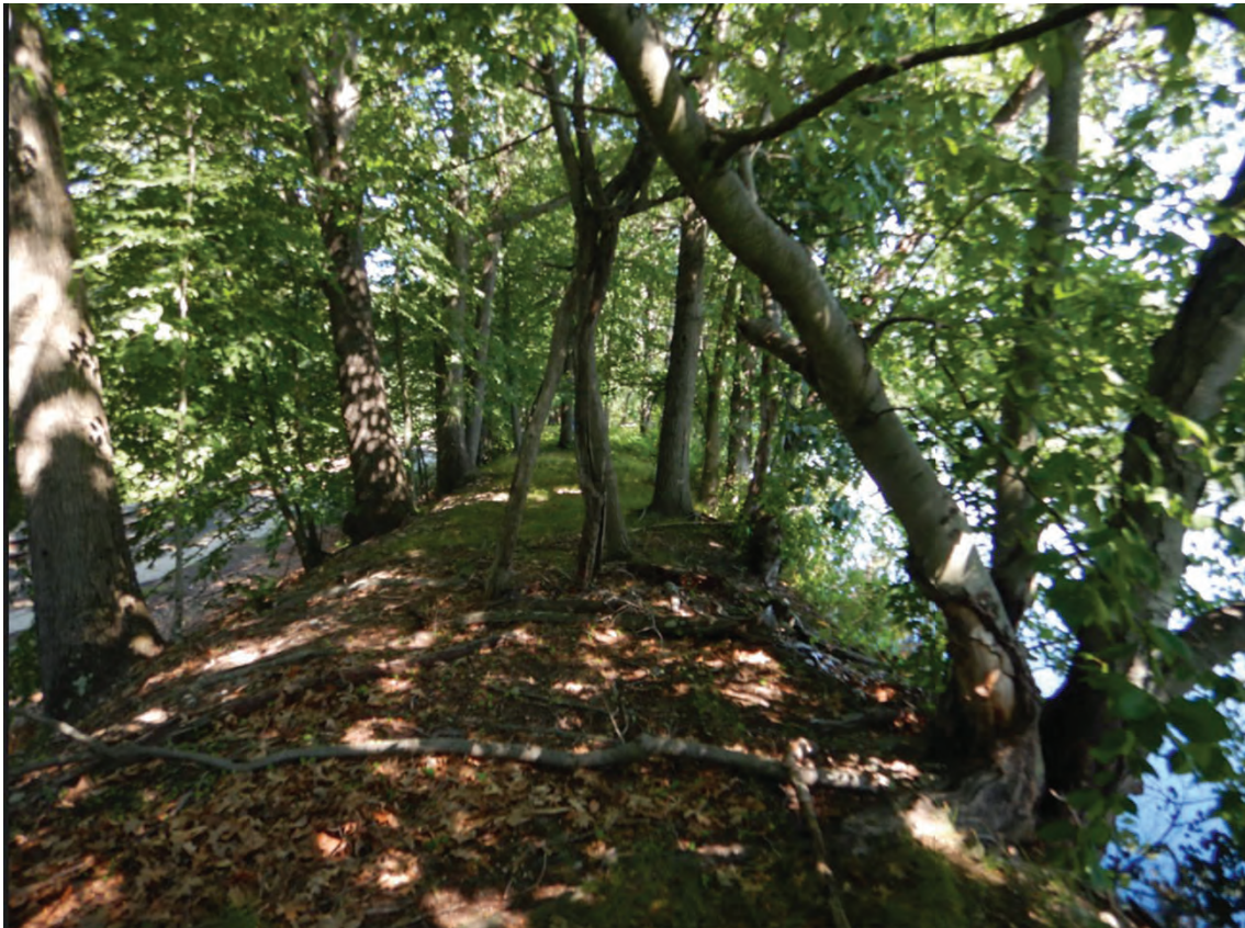
Photo 1: Woody vegetation along the canal embankment
