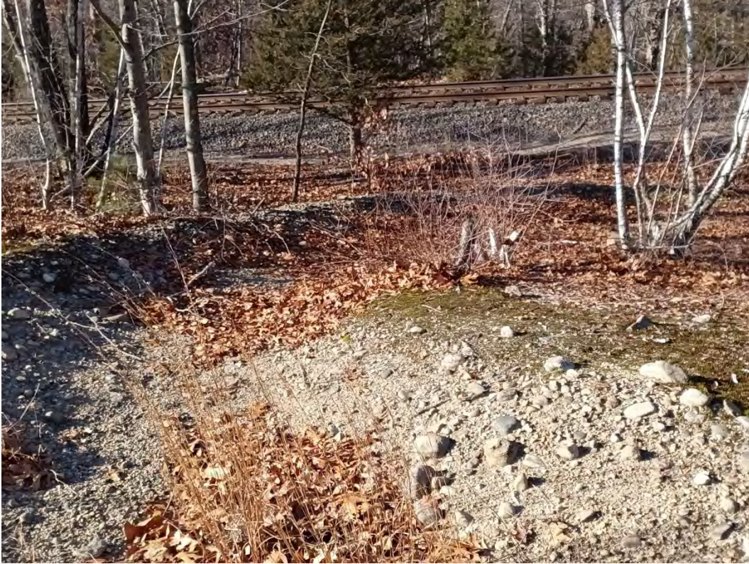
Photo 11. View of Dam Crest. Note Erosion Gully and Gravel
