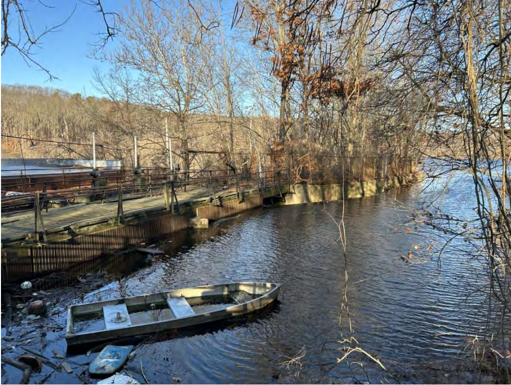
Photo 30. View of Intake Area at Ansonia Powerhouse. Note Trashracks at Intakes
