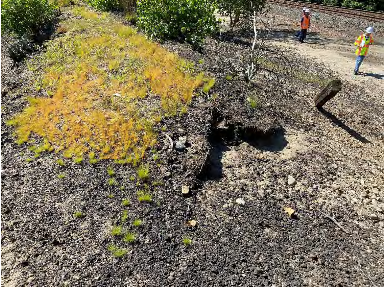
Photo 10- Erosion and rutting in the dam crest
