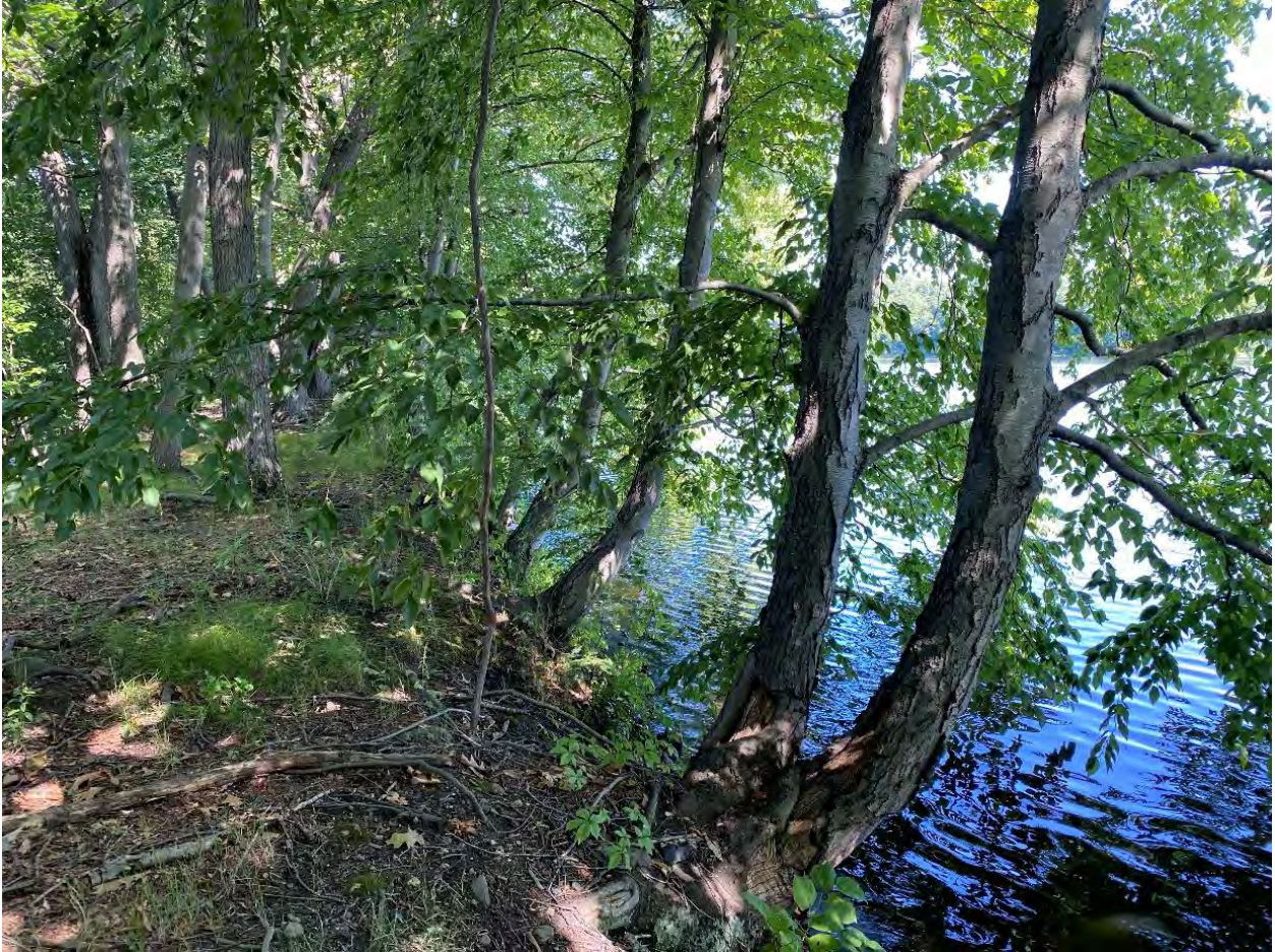
Photo 8- Erosion of the upstream slope, large trees along the water line and across the dam crest
