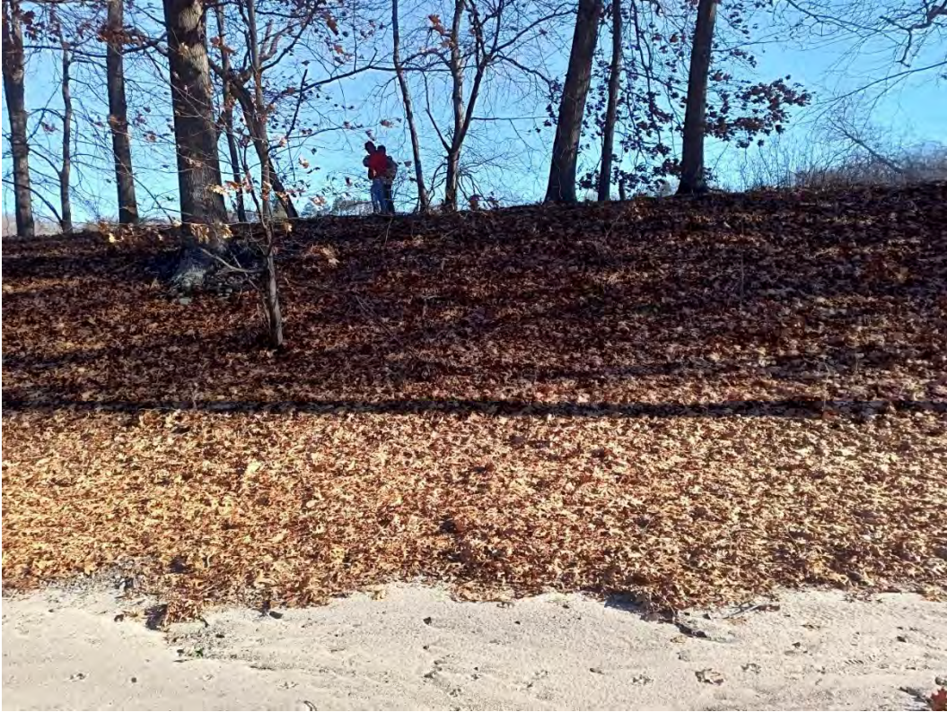
Photo 9. View of Dam Crest. Note Varied Vertical Alignment
