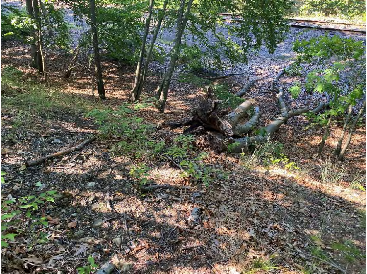
Photo 6- Trees and down trees on the downstream slope near the tracks
