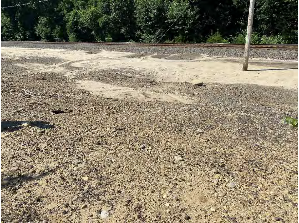
Photo 9- Evidence of water at the toe of the dam next to the railroad tracks.
