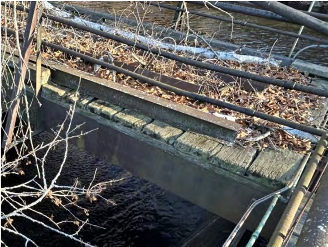
Photo 31. View of Deteriorated Decking
