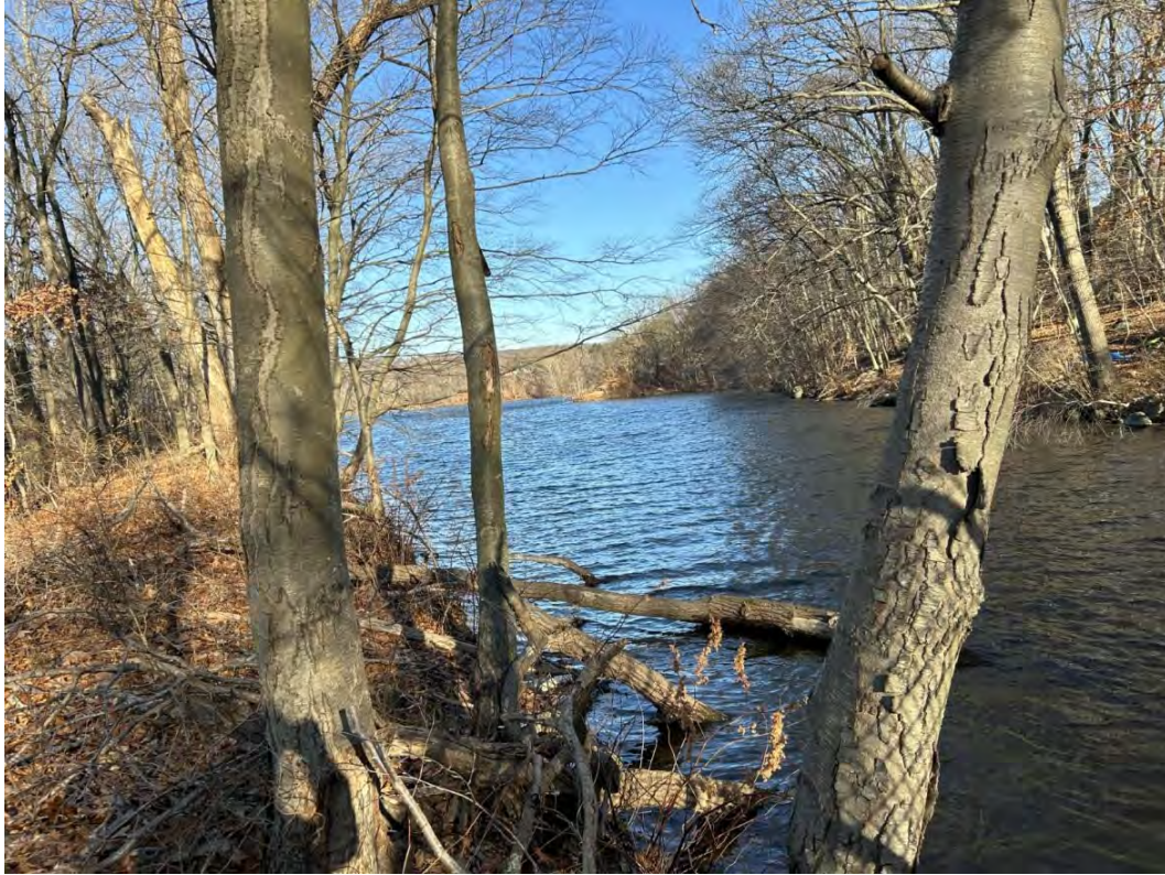
Photo 7. View Inboard Slope of Embankment Dam. Note Large Diameter Trees
