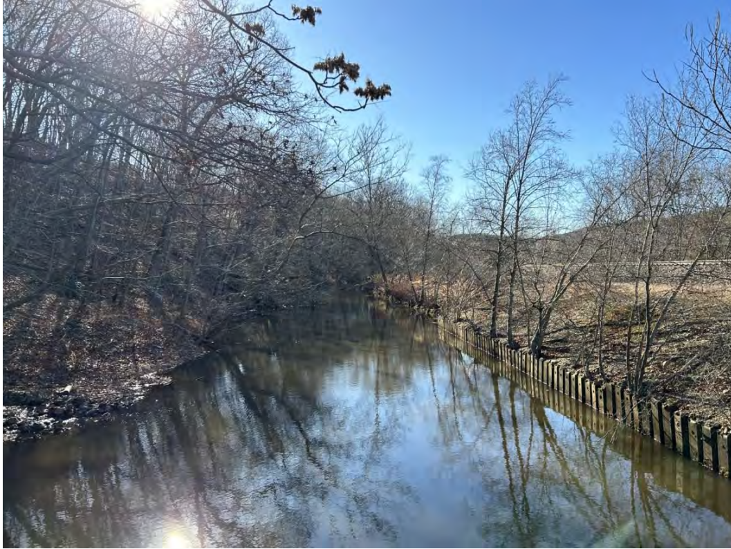
Photo 44. View of Power Canal. Looking Downstream from Gatehouse. Note Sheetpile Retaining Wall
