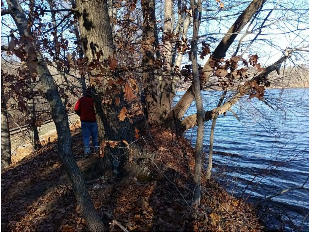
Photo 5. View of Tree on Narrow Section of Embankment Crest (Approximately 14 Feet Wide)
