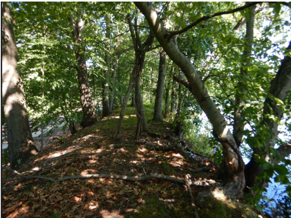
Photo 1: Woody vegetation along the canal embankment
