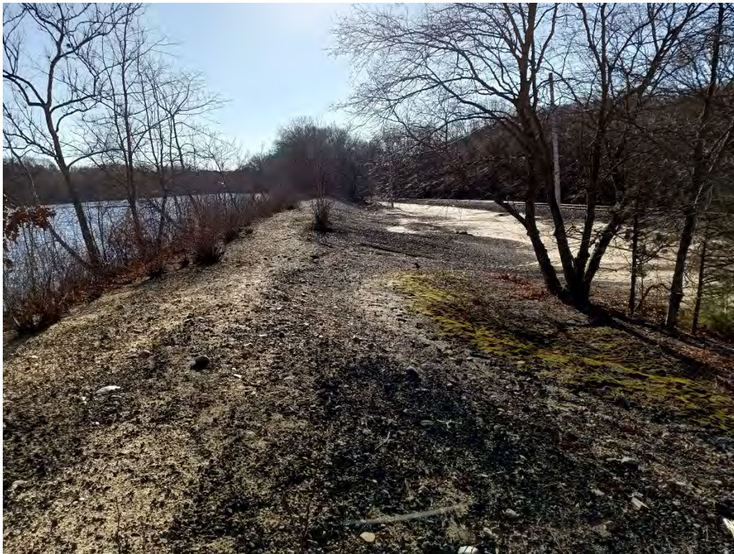
Photo 10. View of Dam Crest. Note Inconsistent Horizontal Alignment
