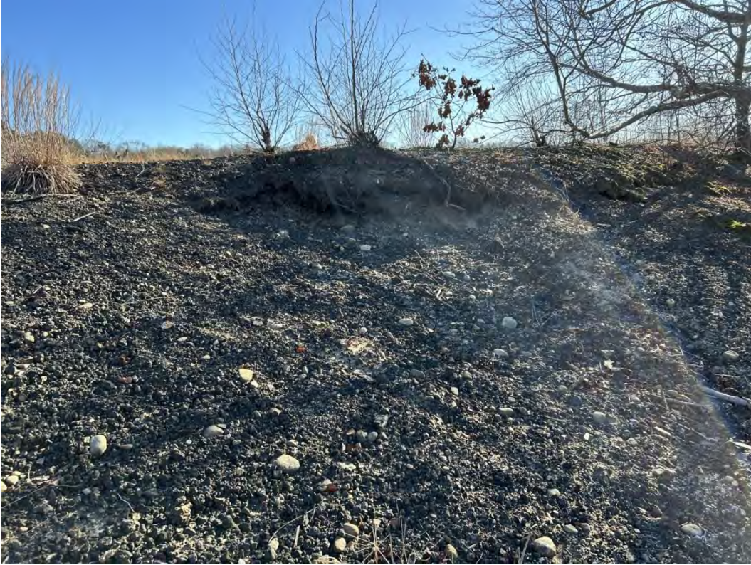
Photo 22. View of Outboard Slope. Note Surface Erosion and Lack of Healthy Vegetation
