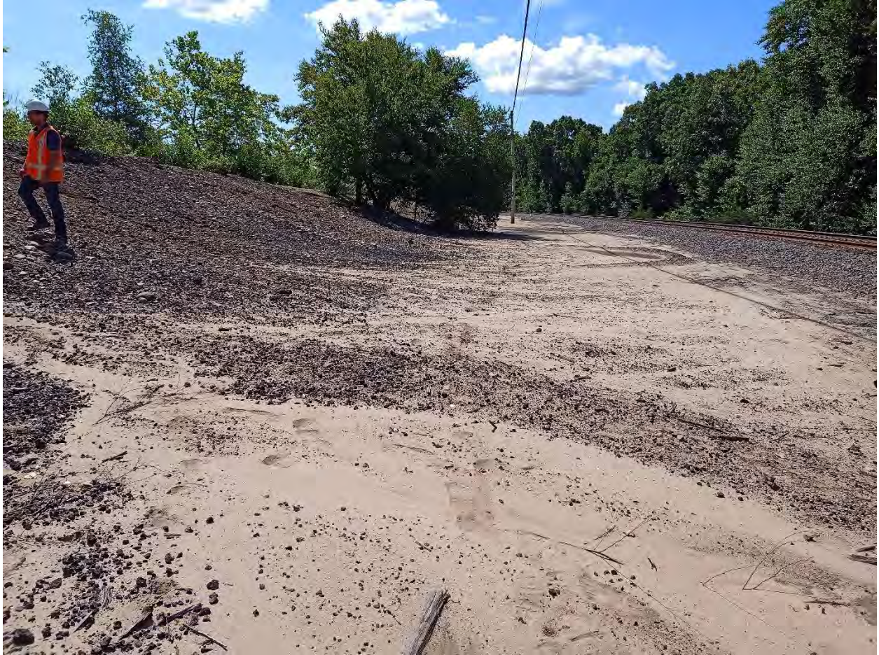
Photo 2-Toe of embankment with accumulated sediment.
