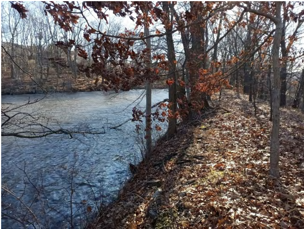
Photo 8. View of Dam Crest and Inboard Slope. Note Steepness of Bank and Large Diameter Trees
