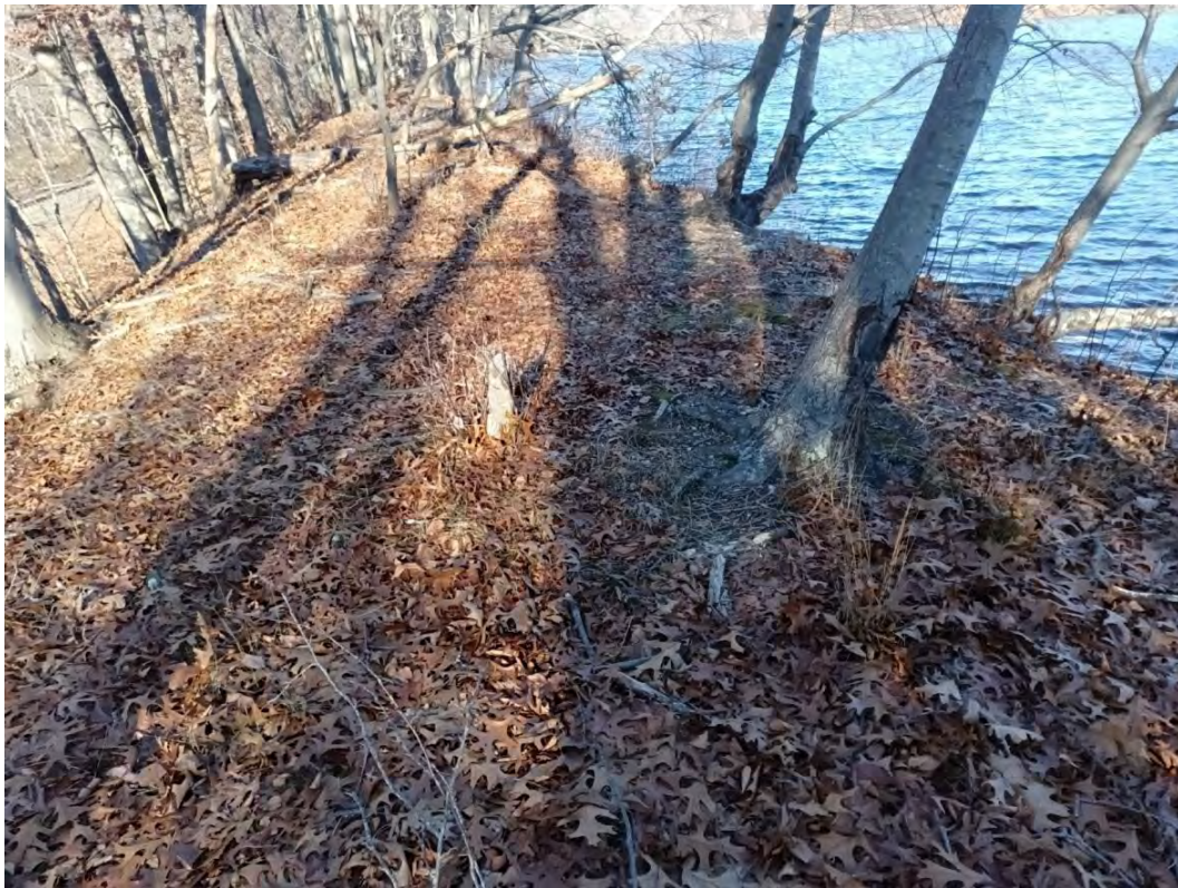
Photo 6. View of Dam Crest. Note Large Diameter Trees and Woody Vegetation
