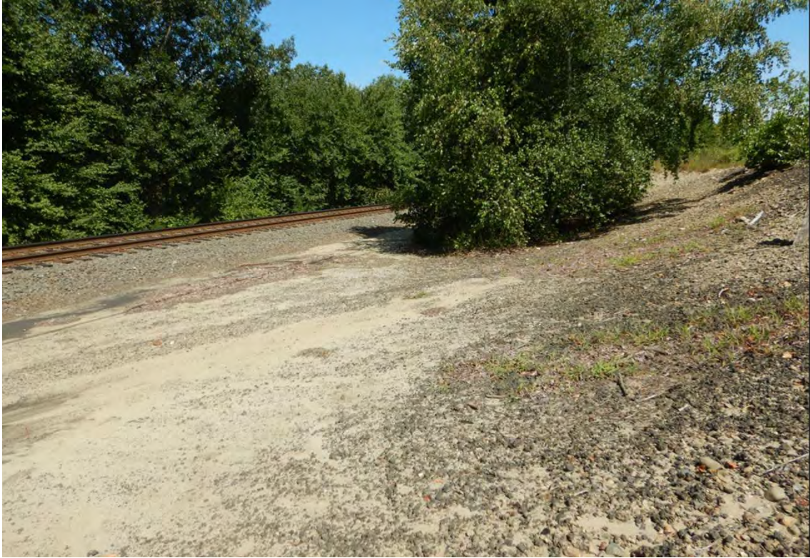
Photo 3: Evidence of washout and possible overtopping of the canal embankment
