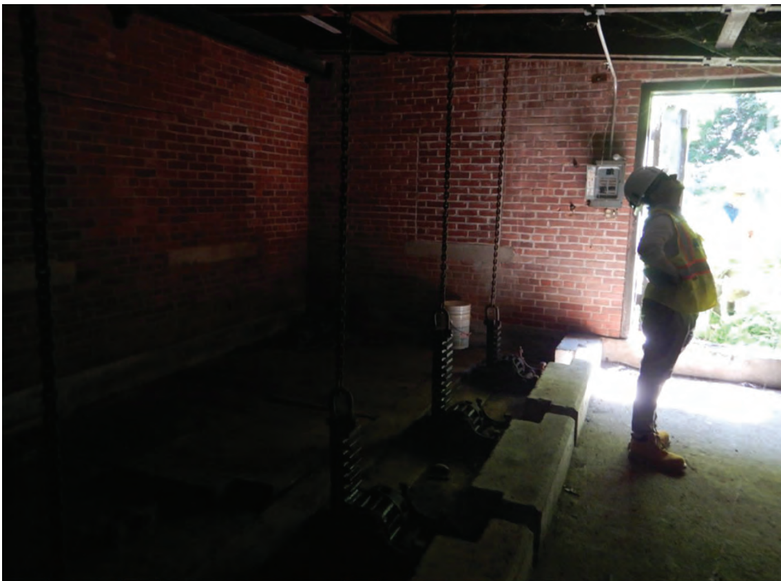
Photo 2: 3 of the 5 gates stuck partially open seen from inside the gatehouse
