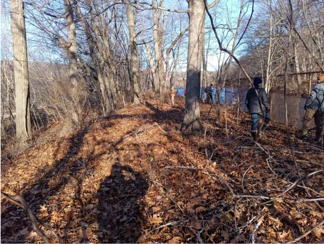
Photo 3. View of Embankment Crest and Outboard Slope of Dam. Note Large Diameter Trees
