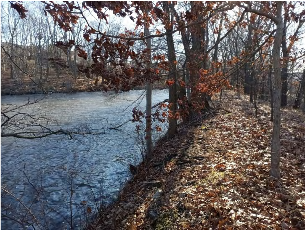
Photo 4. View of Embankment Crest. Note Near Vertical Bank to Water
