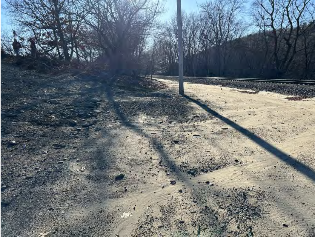
Photo 20. View of Outboard Slope. Note Heavy Vegetation Beyond, and Erosion Rills in Foreground
