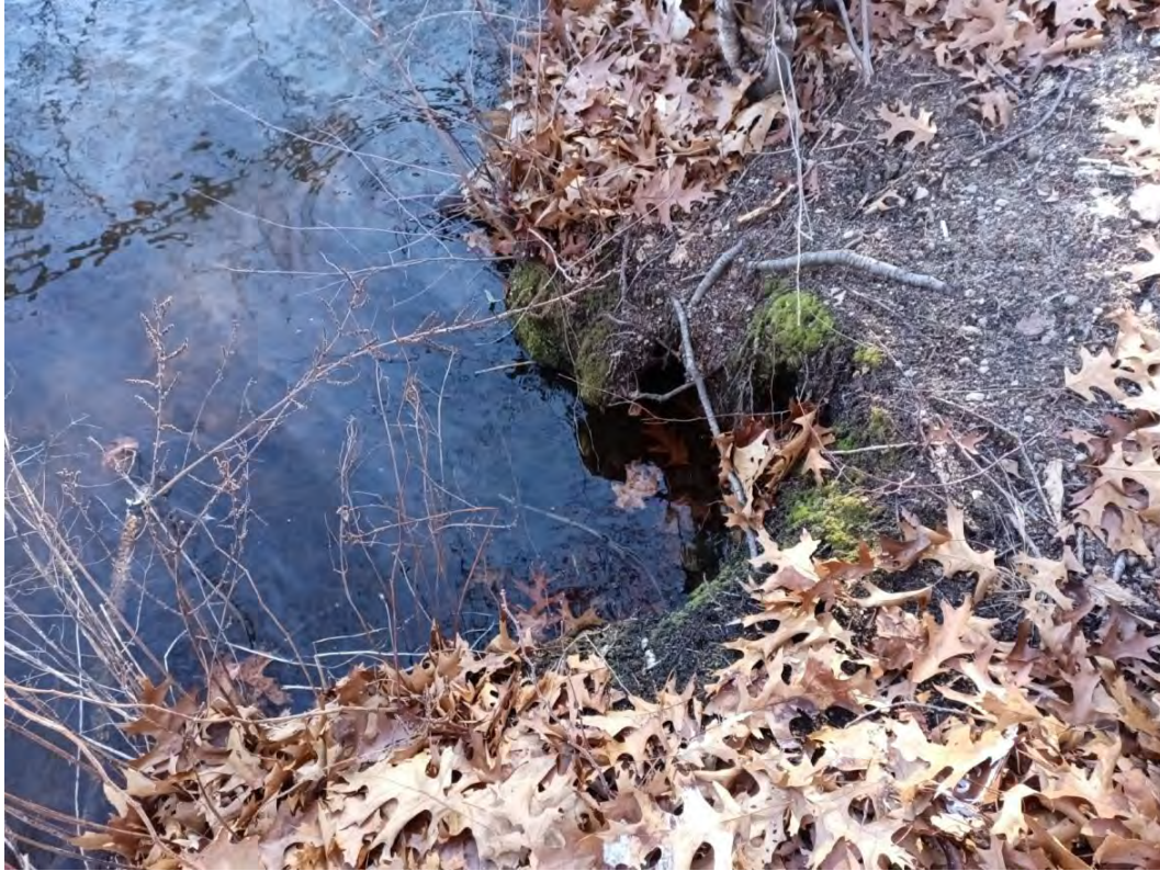
Photo 13. View of Inboard Slope. Note Woody Vegetation and Apparent Rodent Burrow
