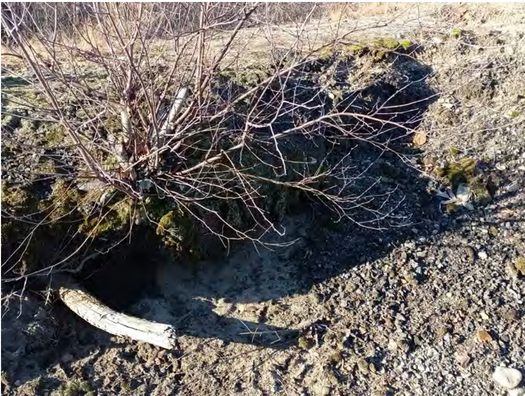
Photo 16. View of Inboard Slope with Erosion Due to Wave Action
