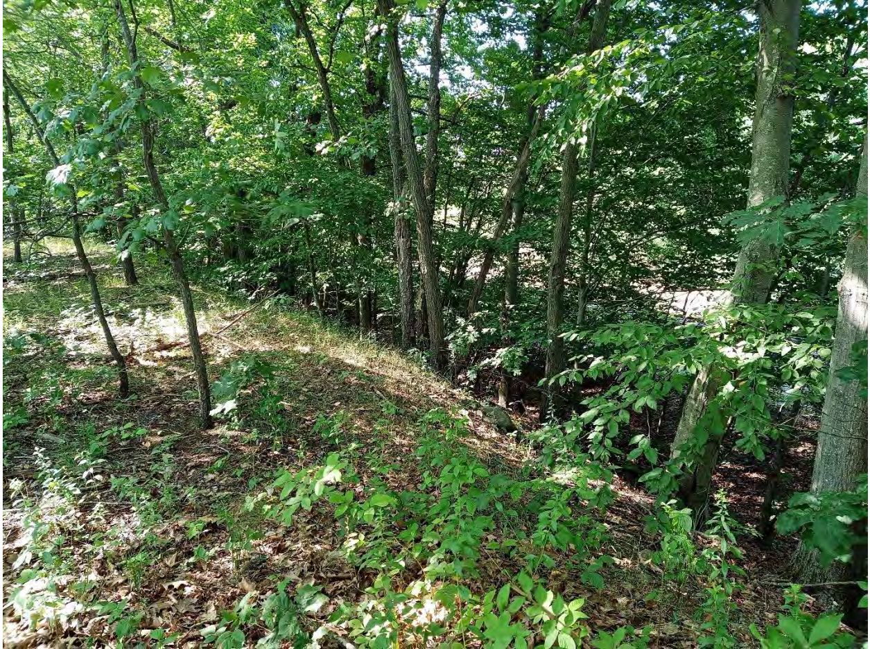
Photo 1-Crest of the dam is overgrown with trees and other woody vegetation.
