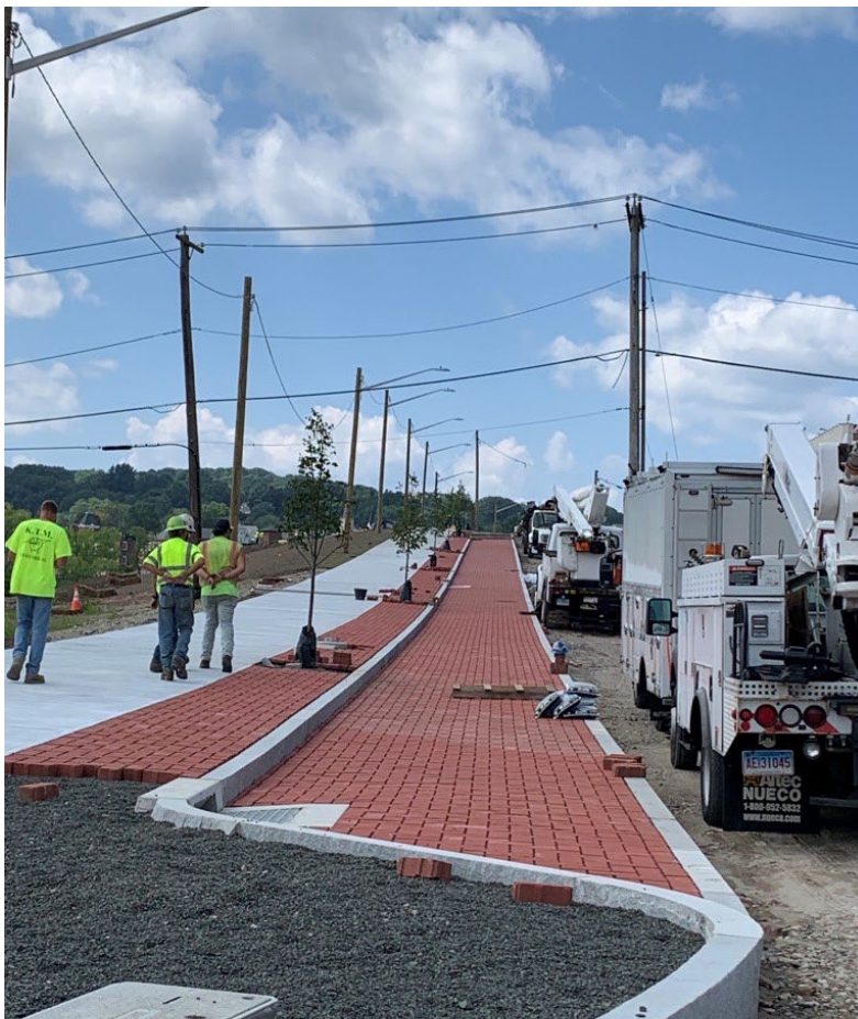
Figure 5 Construction continues along Main Street (Route 34) in Derby. The finished project will include permeable pavers within the parking lane, ADA compliant sidewalks, and pedestrian amenities.
