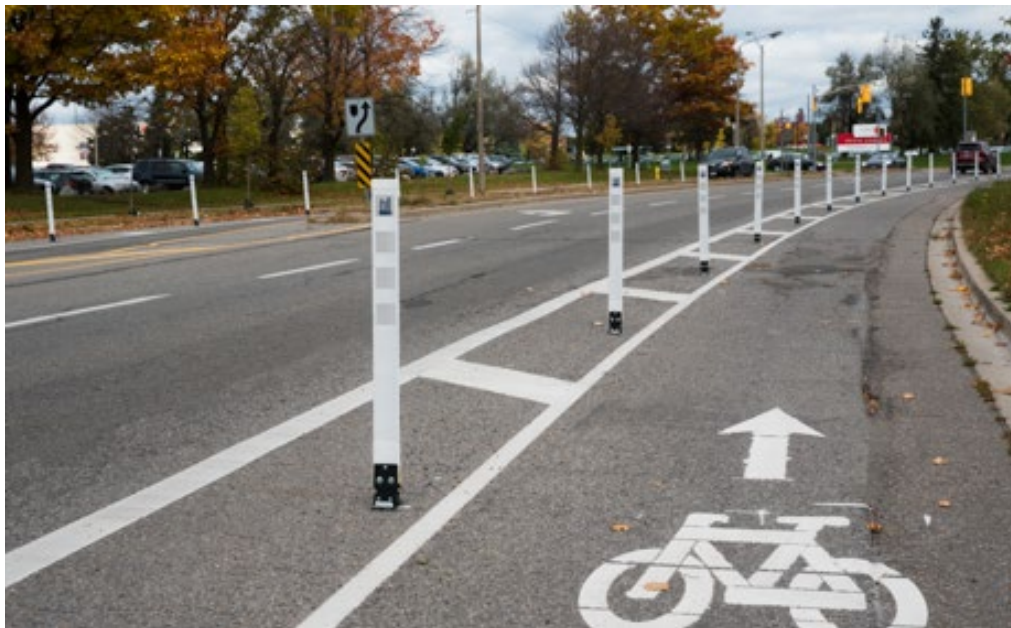
Figure 10 Example of a protected cycle track, using flex posts as buffers.
