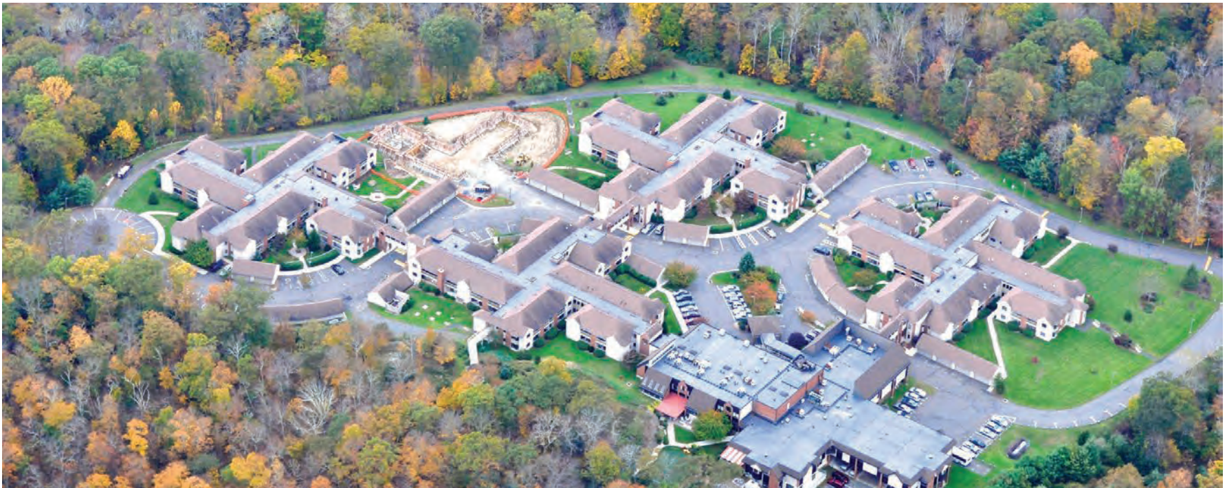
▲ Aerial of Watermark at East Hill [DA]
