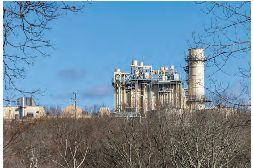
▼ CPV Towantic Energy Center Power Plant in Oxford
