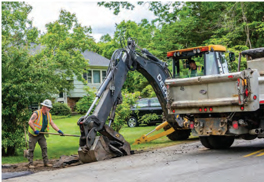
▲ Southbury Public Works
