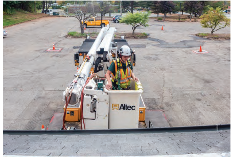
▲ Southbury Public Works
