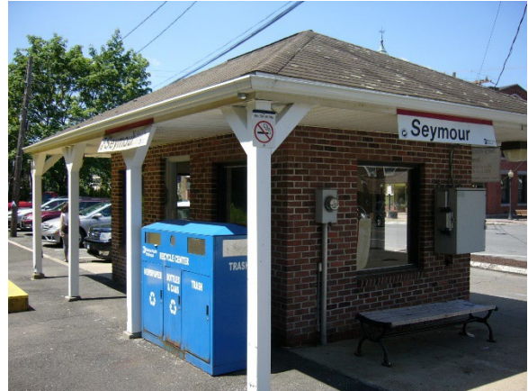
Figure 10 The small structure at the Seymour Train Station
