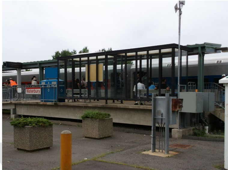
Figure 7 Platform at the Waterbury Train Station
