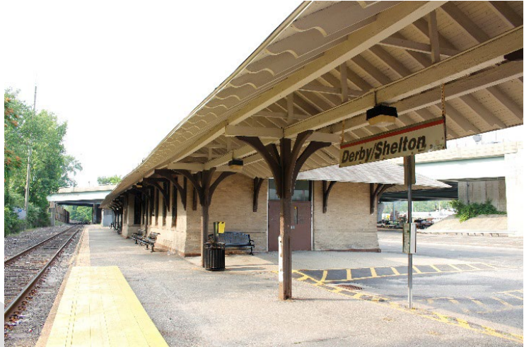
Figure 12 Platform of the Derby-Shelton Train Station looking south
