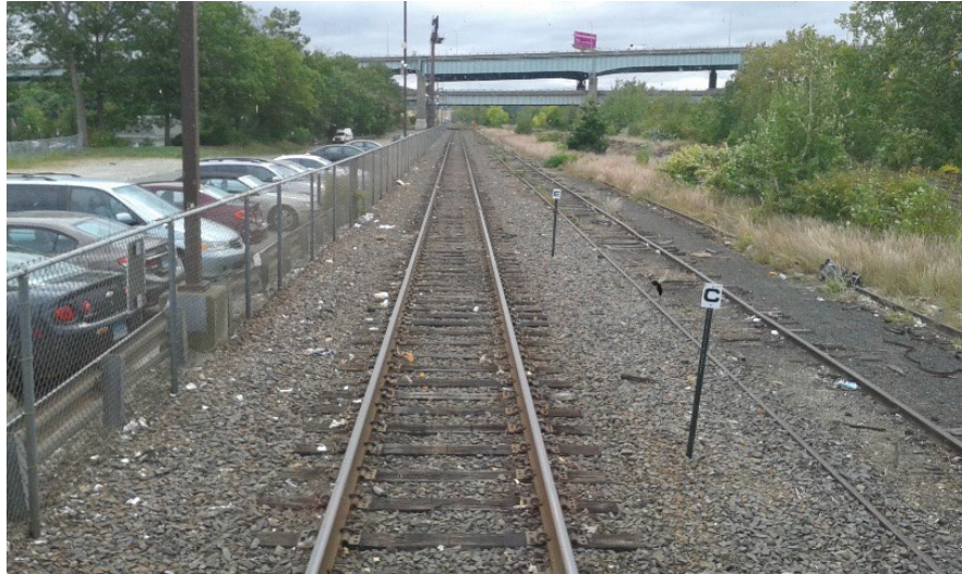
Figure 6 View southbound from the Waterbury Train Station
