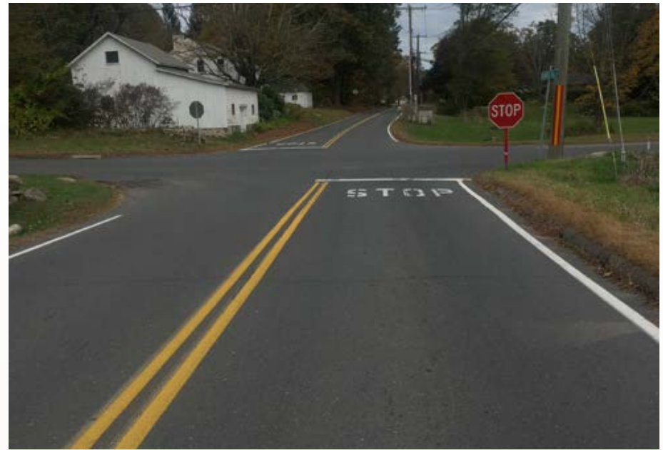
Talmadge Hill Rd/Matthew Rd/ CT-68 (Cheshire Rd)
