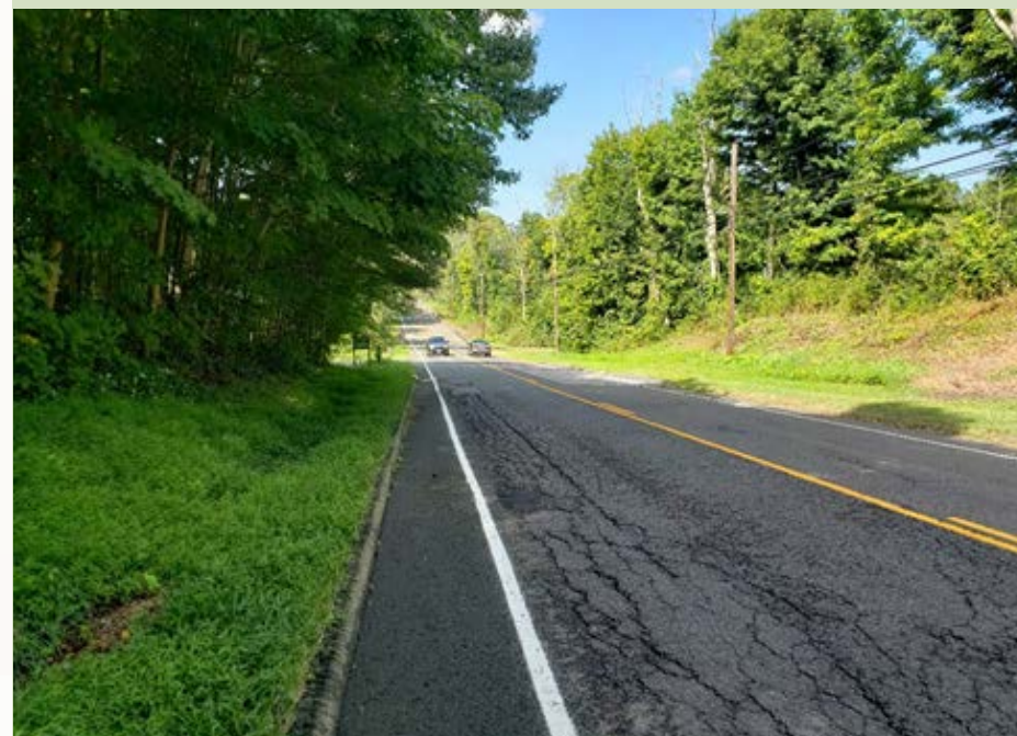
CT-132 (Kasson Rd) looking west from Woodland Rd
