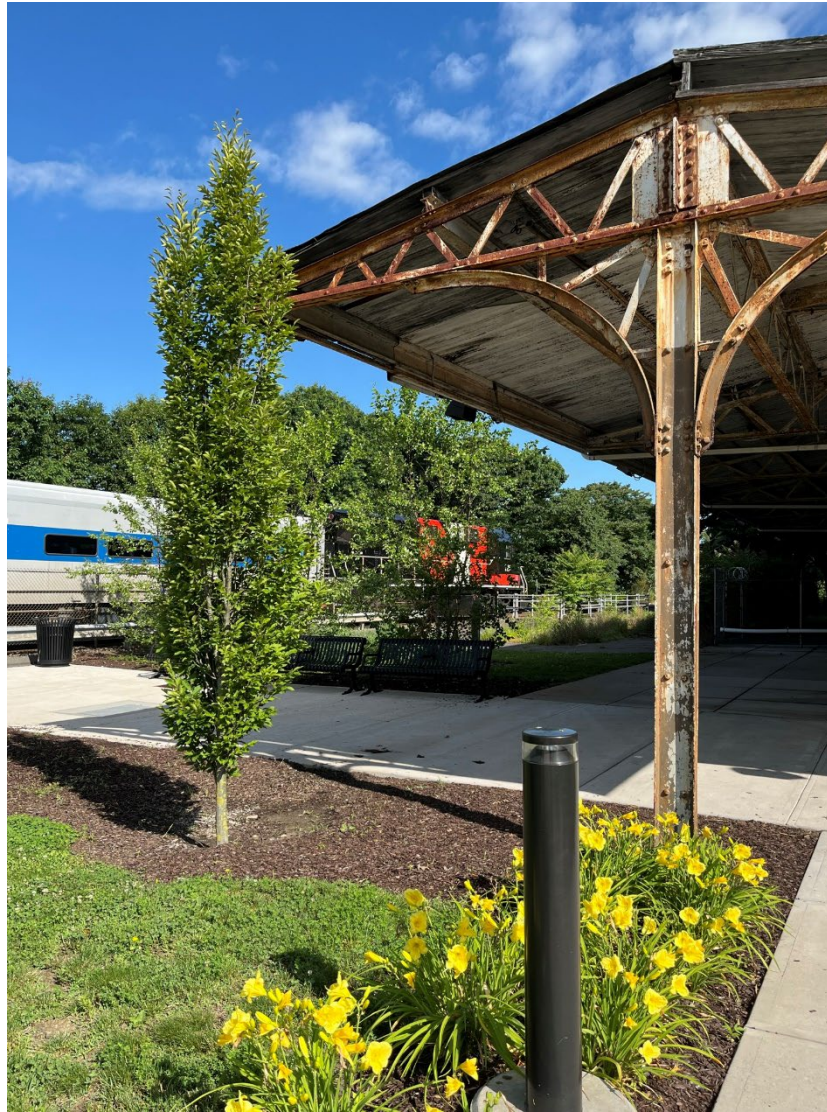
Figure 4 Waterbury Line train stopped at the Waterbury station
