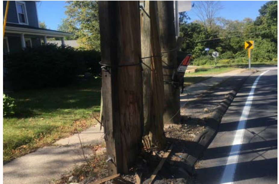
Utility poles on US-6 (Main St) along horizontal curvature
