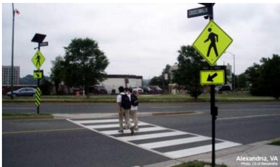
Picture of RRFB Installation (NACTO / City of Alexandria, VA)
