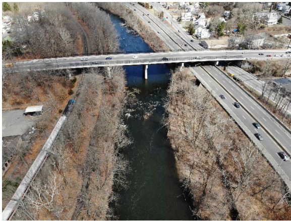
Figure 2 The Waterbury Line and Route 8 run alongside the Naugatuck River under the Prospect Street Bridge, Naugatuck
