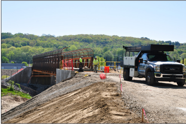
Prefabricated pedestrian bridges like the one installed over the Waterbury Rail Line in Ansonia are popular due to decreased construction timelines and cost compared to bridges constructed on site.
