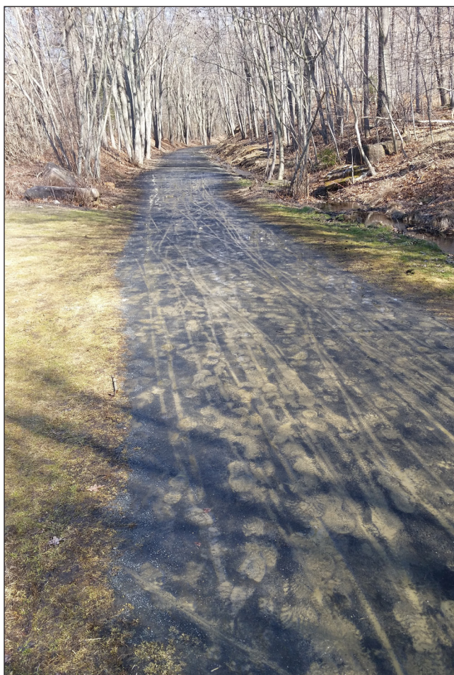
Compacted stone dust trails can become rutted when wet, and often require more upkeep than paved trails. (Air Line State Park Trail, East Hampton)
