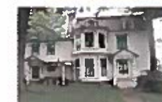
36. Amos Baldwin House , 1800. aka Beadle-Johnson House. 2nd Empire; mansard roof added 1872.
