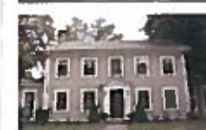
18. Preston/Trythall House , 1828. Colonial Revival conversion 1925 by Alice Washburn (her family home).
