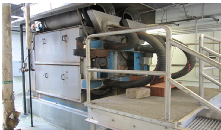
Figure 4-7 Seymour Rotary Drum Thickener
