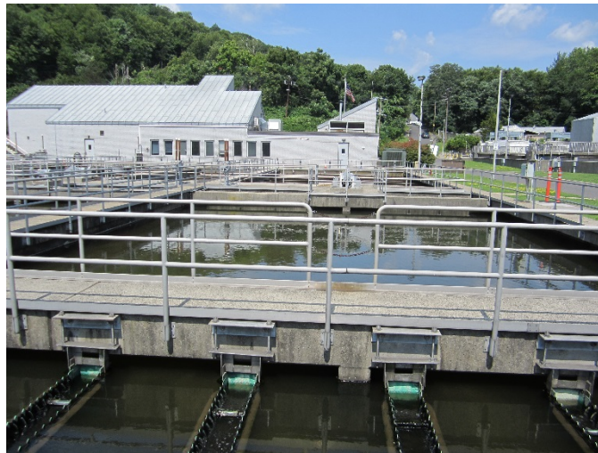
Figure 6-6 Naugatuck Secondary Clarifiers
