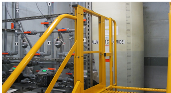
Figure 4-6 Seymour Alum Feed System for P Removal
