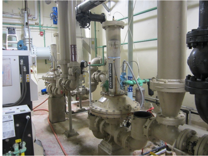
Figure 3-4 Ansonia Sludge Pumps
