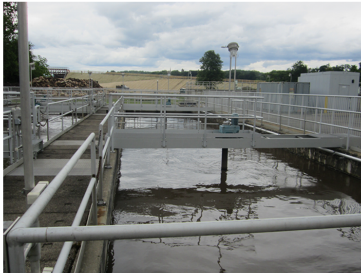
Figure 3-5 Ansonia Converted Anoxic Basins
