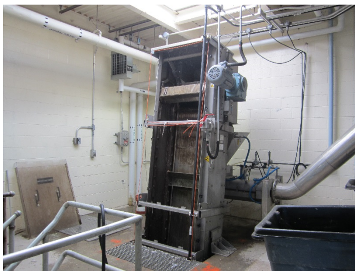
Figure 3-1 Ansonia Mechanical Bar Screen
