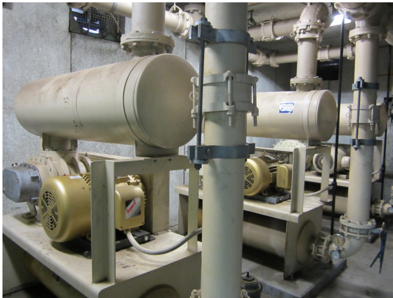
Figure 5-5 Beacon Falls Aeration Blowers
