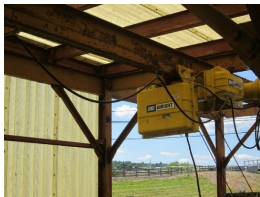
Figure 2-3 Derby Grit Facility Overhead Clamshell Hoist
