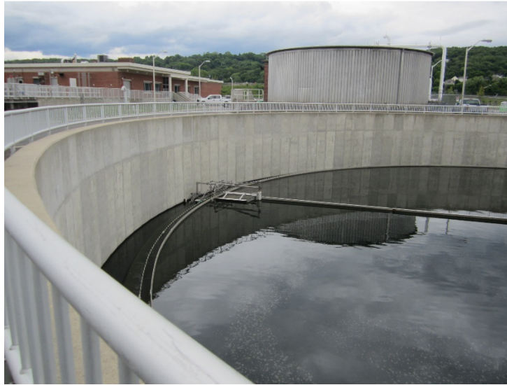
Figure 3-7 Ansonia Secondary Clarifier
