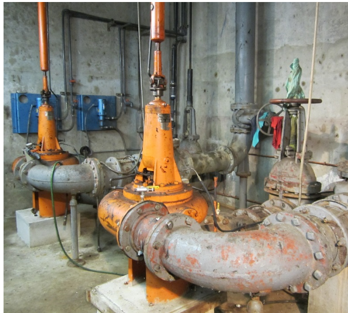
Figure 2-2 Derby Influent Pumps with Extended Shafts
