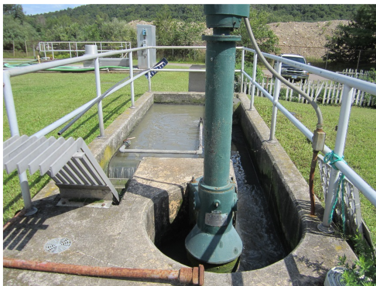
Figure 5-2 Beacon Falls Comminutor and Bar Screen
