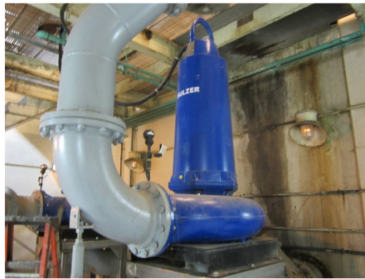
Figure 6-1 Naugatuck New Sulzer Influent Pump
