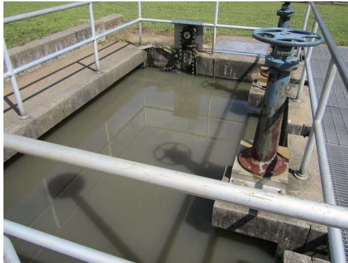
Figure 5-3 Beacon Falls Rectangular Primary Clarifier
