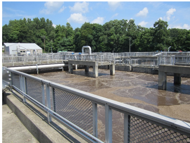
Figure 6-4 Naugatuck Activated Sludge Aeration Basin
