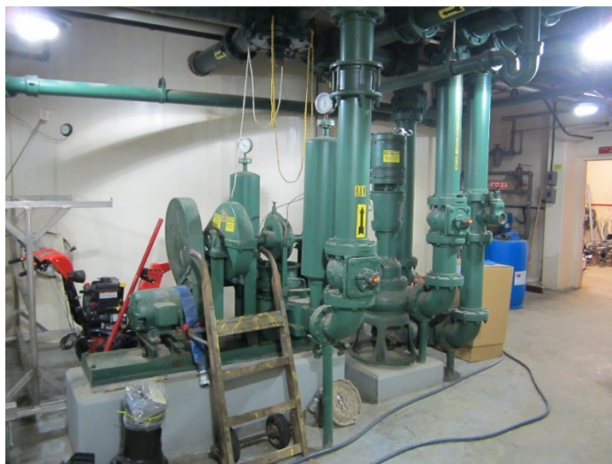
Figure 5-8 Beacon Falls Plunger Pumps for Sludge
