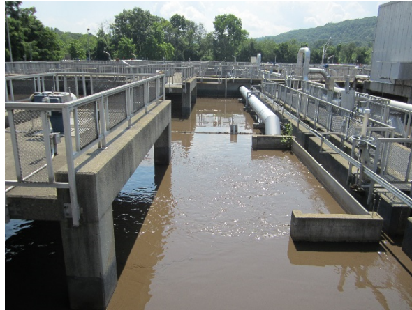
Figure 6-3 Naugatuck Anoxic Basins, in Modified 4-Stage Bardenpho Process
