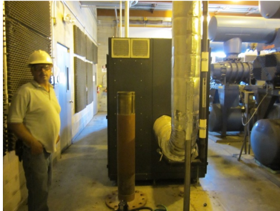
Figure 6-5 Naugatuck Piller Turbo Blower, for Aeration System
