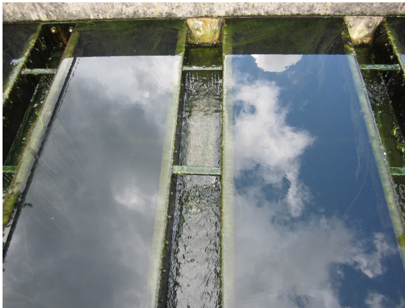
Figure 5-6 Beacon Falls Secondary Clarifier Effluent Weirs
