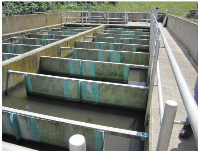
Figure 2-9 Derby Chlorine Contact Basins
