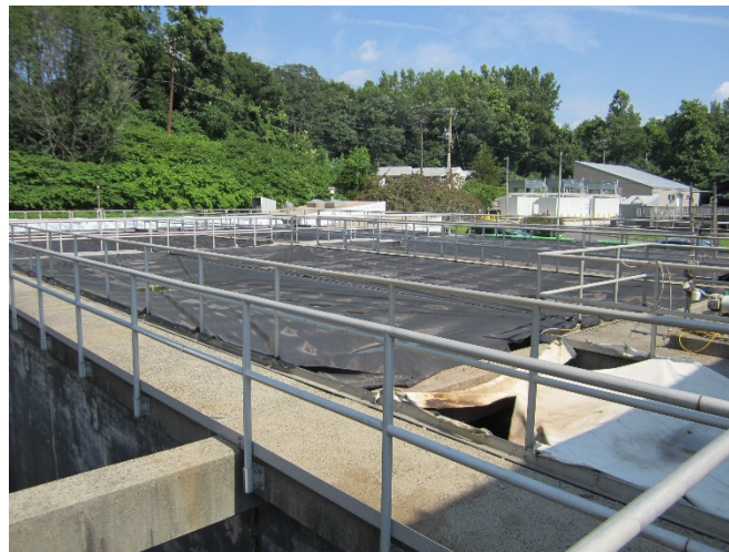
Figure 6-2 Naugatuck Primary Settling Tanks, Covered for Odor Control
