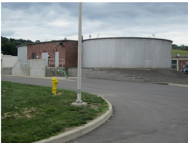
Figure 3-9 Ansonia Former Digesters Used for Sludge Storage
