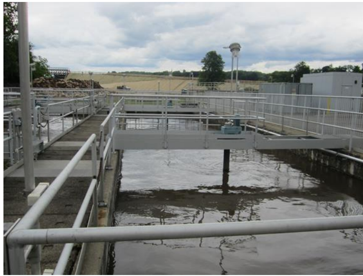
Figure 3-5 Ansonia Converted Anoxic Basins
