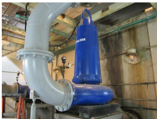
Figure 6-1 Naugatuck New Sulzer Influent Pump
