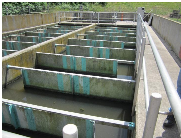
Figure 2-9 Derby Chlorine Contact Basins
