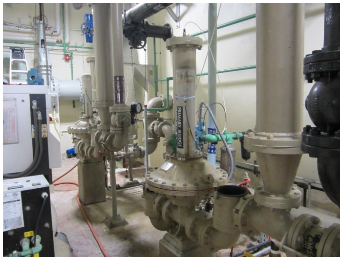
Figure 3-4 Ansonia Sludge Pumps
