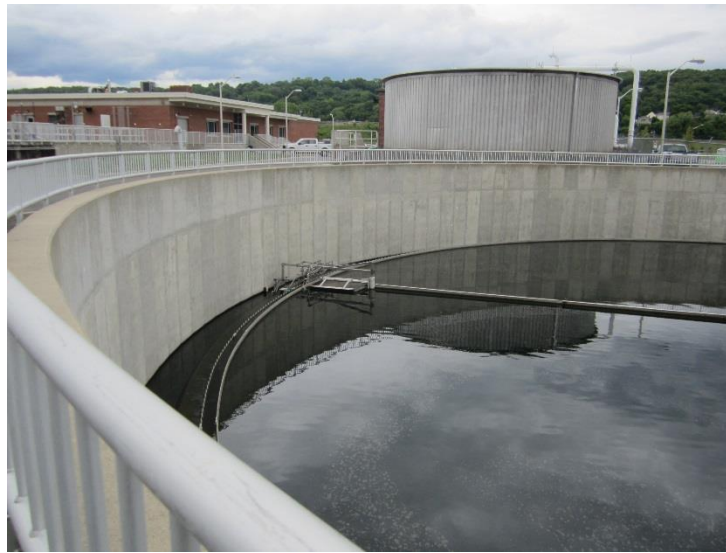
Figure 3-7 Ansonia Secondary Clarifier
