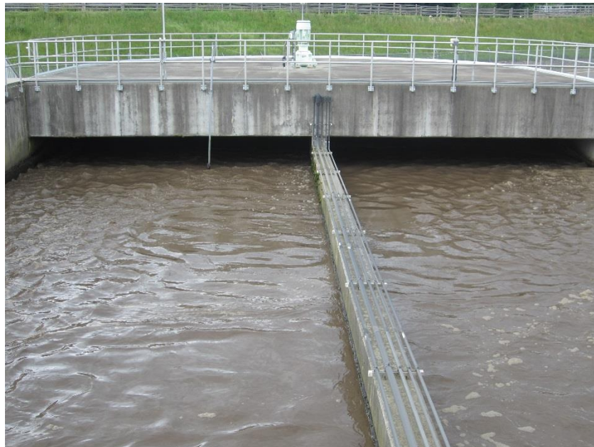
Figure 3-6 Ansonia Oxidation Ditch Aeration Basin
