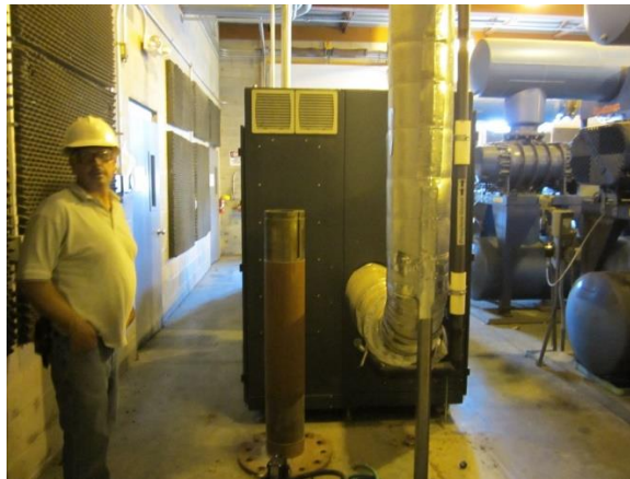
Figure 6-5 Naugatuck Piller Turbo Blower, for Aeration System
