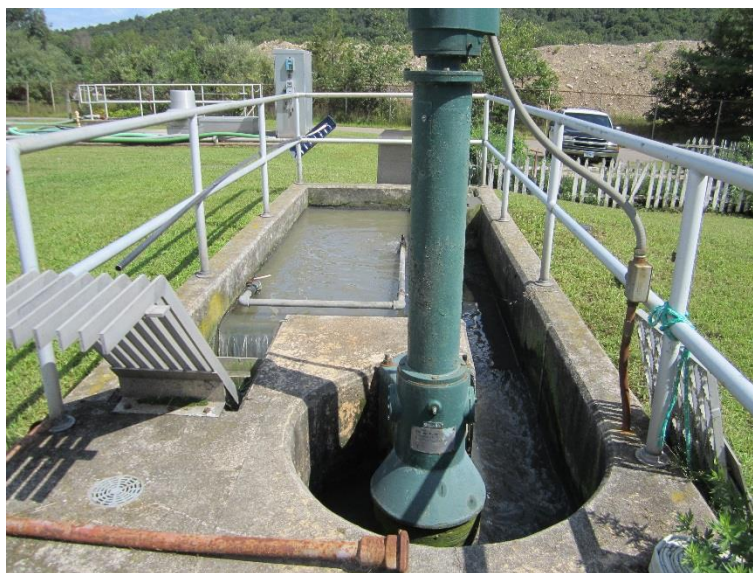
Figure 5-2 Beacon Falls Comminutor and Bar Screen
