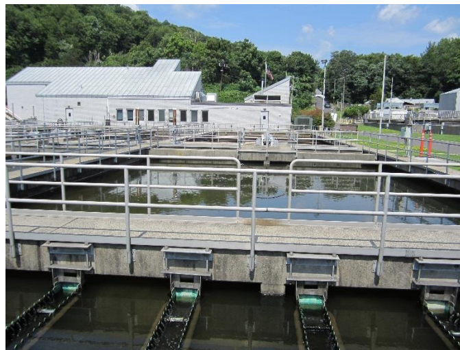
Figure 6-6 Naugatuck Secondary Clarifiers
