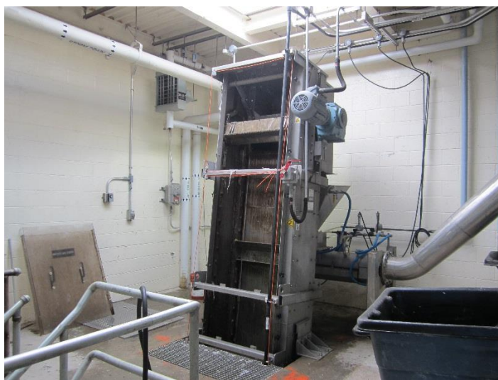
Figure 3-1 Ansonia Mechanical Bar Screen
