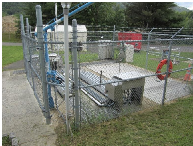
Figure 5-7 Beacon Falls UV Disinfection System
