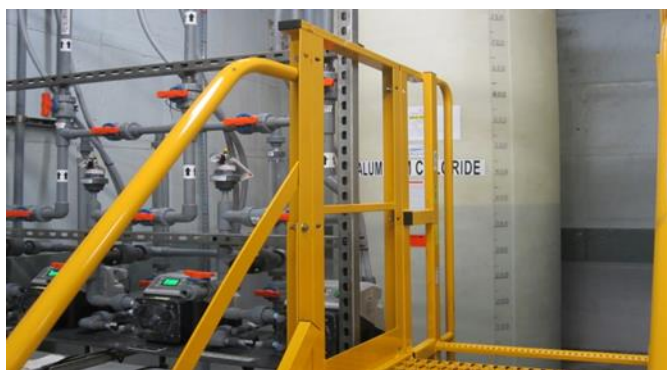
Figure 4-6 Seymour Alum Feed System for P Removal
