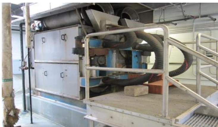
Figure 4-7 Seymour Rotary Drum Thickener
