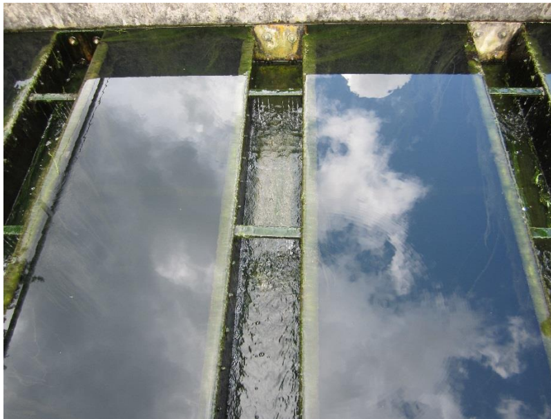
Figure 5-6 Beacon Falls Secondary Clarifier Effluent Weirs
