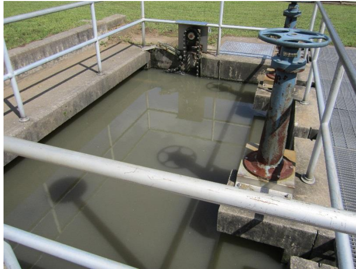
Figure 5-3 Beacon Falls Rectangular Primary Clarifier
