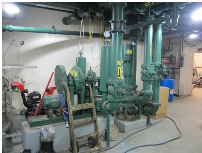
Figure 5-8 Beacon Falls Plunger Pumps for Sludge
