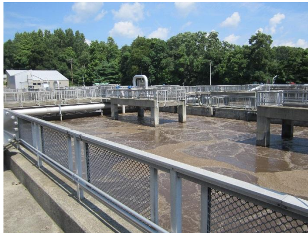
Figure 6-4 Naugatuck Activated Sludge Aeration Basin
