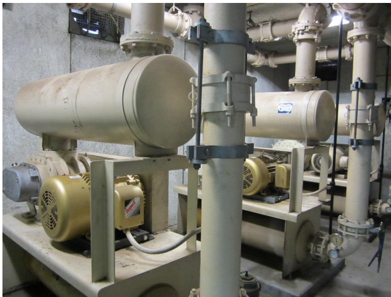
Figure 5-5 Beacon Falls Aeration Blowers
