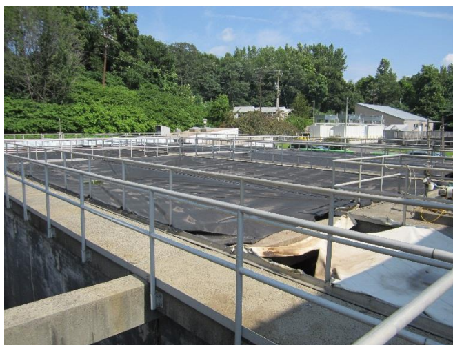
Figure 6-2 Naugatuck Primary Settling Tanks, Covered for Odor Control
