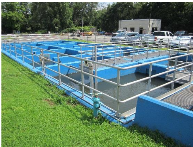
Figure 6-7 Naugatuck Chlorine Contact Basins
