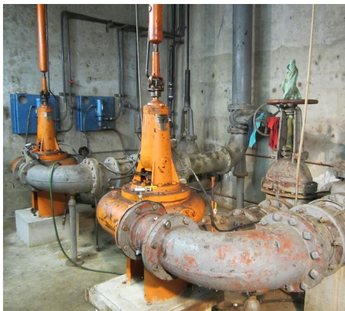
Figure 2-2 Derby Influent Pumps with Extended Shafts
