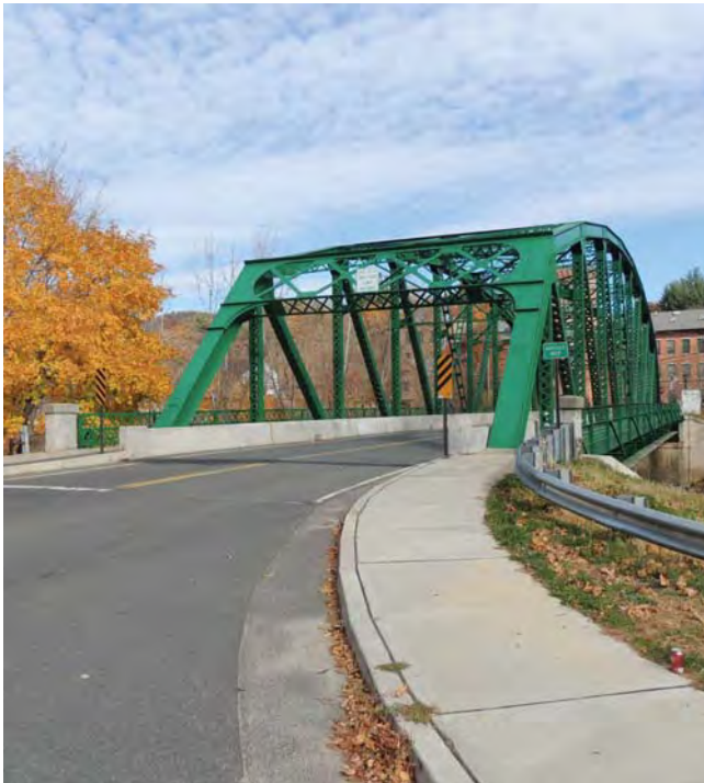
The renovated Depot Street Bridge, Beacon Falls
