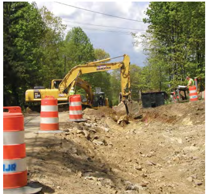
Scott Road Construction, Prospect
