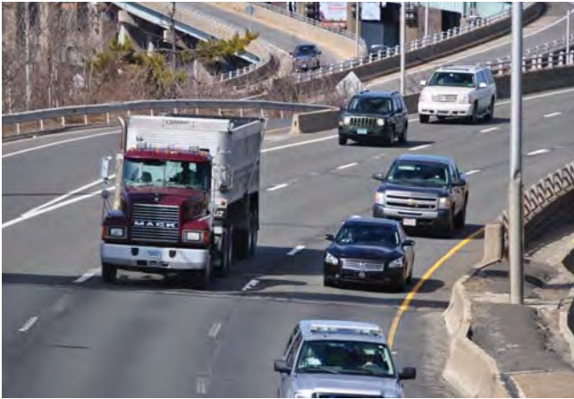
Truck on I-84 eastbound
