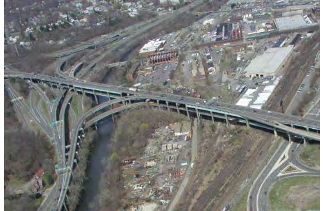
I-84/Rte 8 Interchange, Waterbury, COGCNV Aerial Flight April 2007
