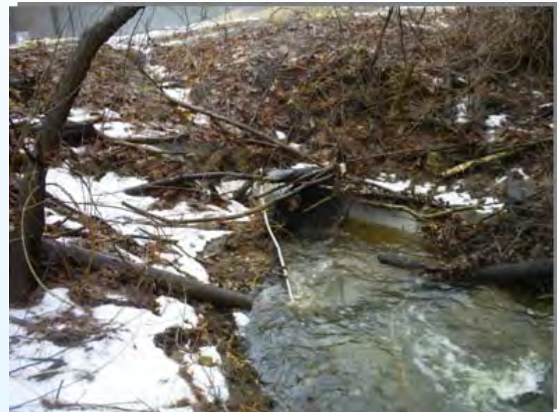
Partially Blocked Culverts Pose Threats During Heavy Rain Storms
