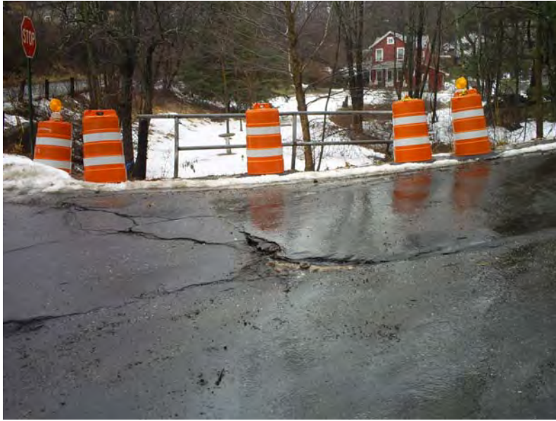
Altair Avenue (bridge concrete peeking through pavement)
