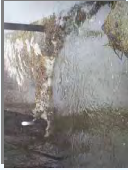
Undersized Culvert @ Hulls Hill Road / Jeremy Swamp Road Intersection
