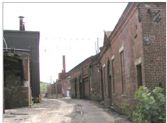
Former Plume & Atwood Brass Mill, Thomaston
