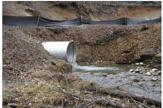
Outfall, Beacon Falls
