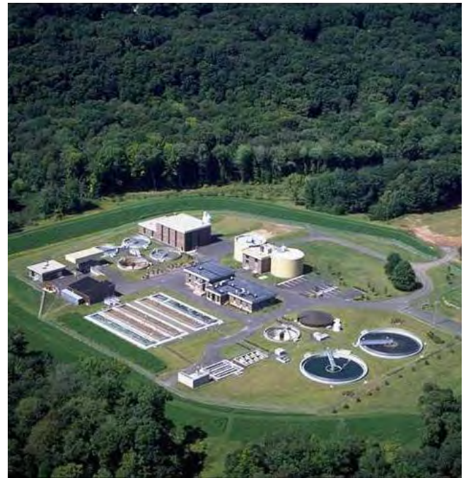
Wastewater Treatment Plant, Cheshire
