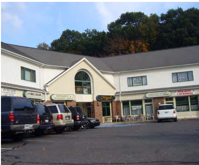
Commercial Buildings, Wolcott
