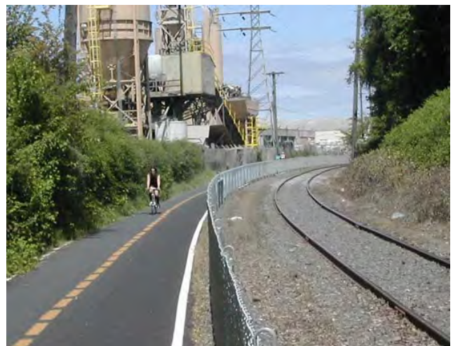
Greenway trail in Portland, Oregon that runs within 10-15' of the centerline of the adjacent active rail line.
