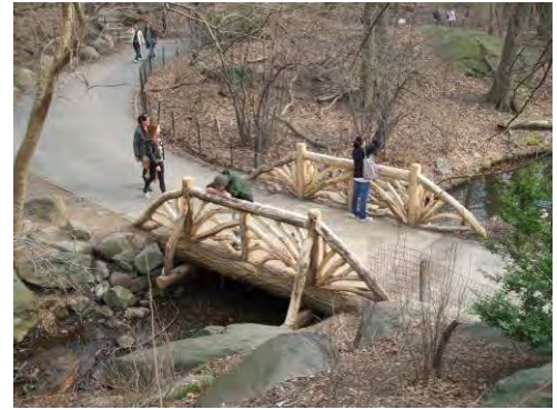
The new bridge over Branch Brook could look similar to some of the rustic examples in Central Park.
