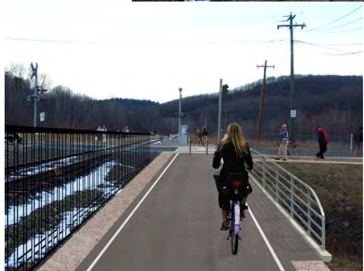
Figure 6: Greenway trail intersection with Frost Bridge Road (Route 262) and the Naugatuck Railroad. Improvements include: a greenway-user activated traffic signal and railroad crossing warning lights, signage and gates.
