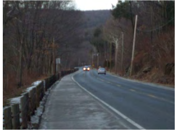
View north along Waterbury Road toward Frost Bridge Road.
