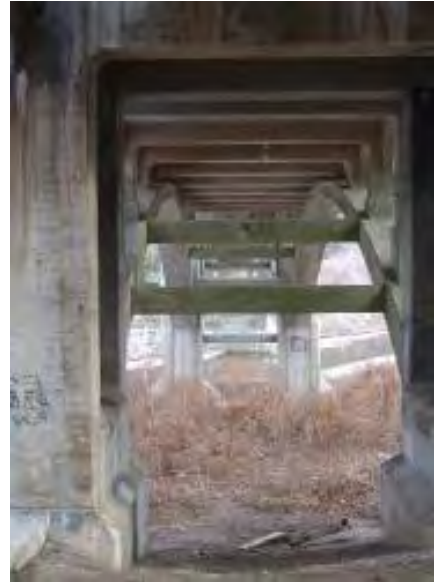
The structural arches below the Reynolds Bridge.
