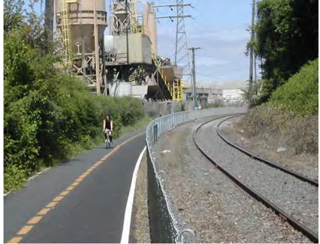
Greenway trail in Portland, Oregon whose edge runs within 10-15' of the centerline of the adjacent active rail line.
