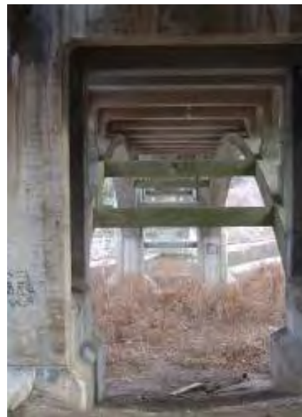
The structural arches below the Reynolds Bridge.
