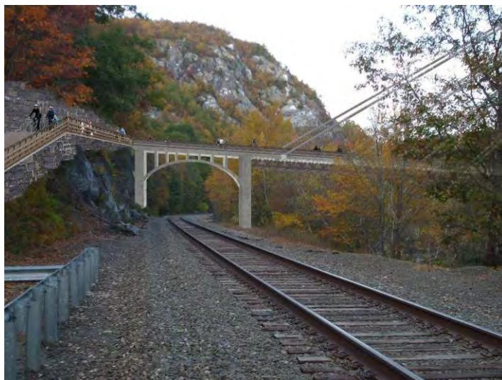
Figure 32: Existing and photo-simulation view of the west end of the long-span bridge over Route 8, the river and the railroad line. The structural piers are configured to accommodate a second track in the future.
