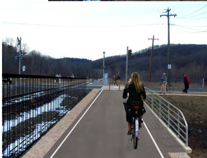
Figure 16: Greenway trail intersection with Frost Bridge Road (Route 262) and the Naugatuck Railroad. Improvements include: a greenway-user activated traffic signal and railroad crossing warning lights, signage and gates.
